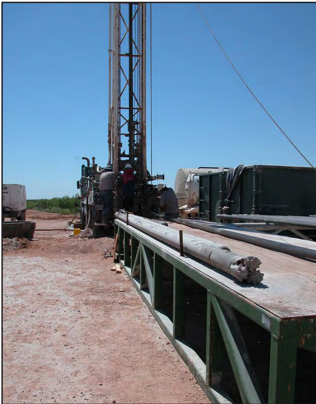
West Texas Water Well Service, Rig #15 at SNL-15, viewed toward the west. The 7.875-inch rotary bit has been laid down, and the crew is tripping in to begin coring using compressed air. Photo taken June 5, 2005, by Dennis W. Powers.
