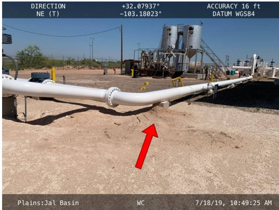
Backfilled Excavation
