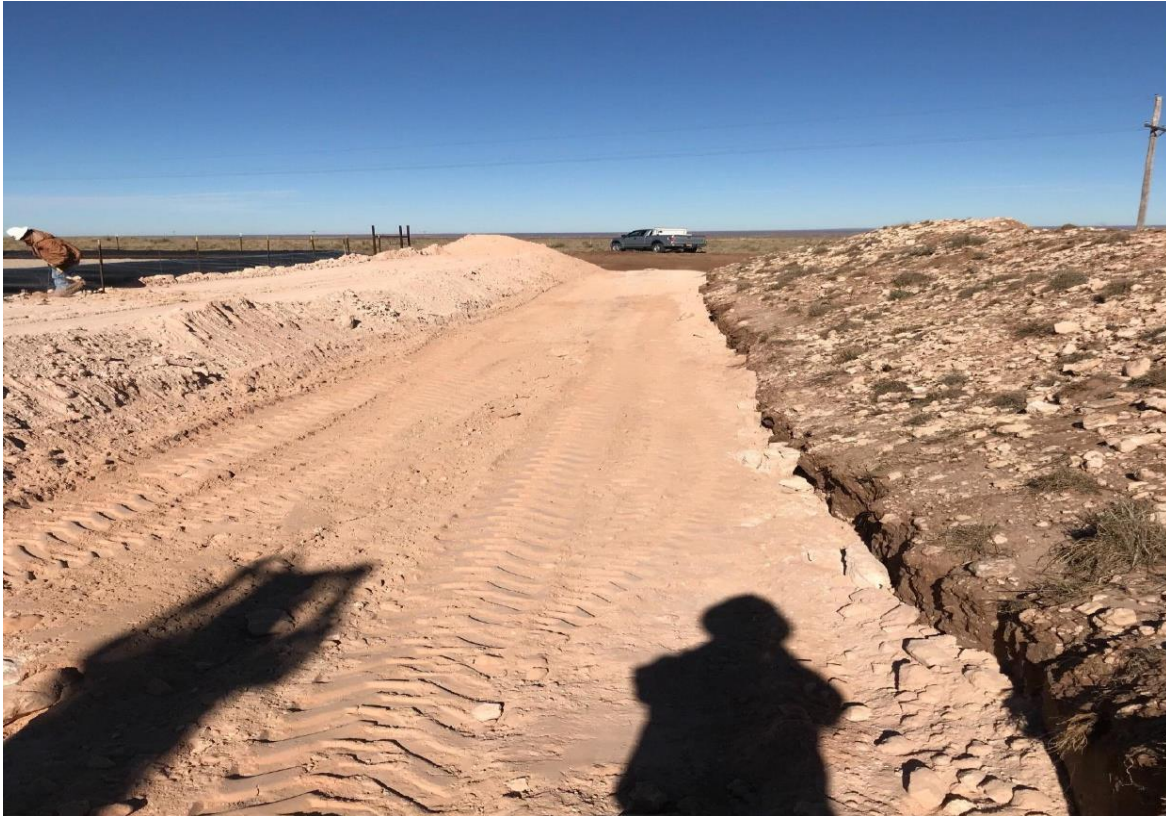
View Northwest, Backfill of Pasture Area
