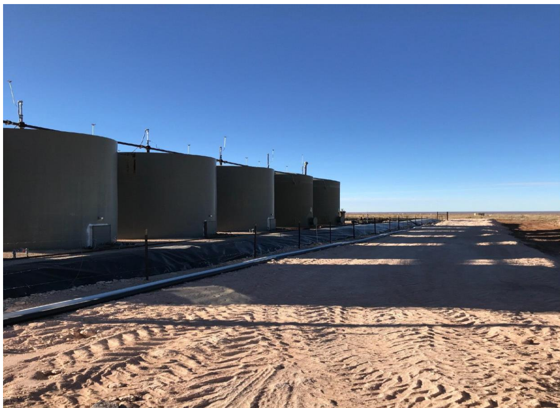
View Southeast, Pad backfill Area
