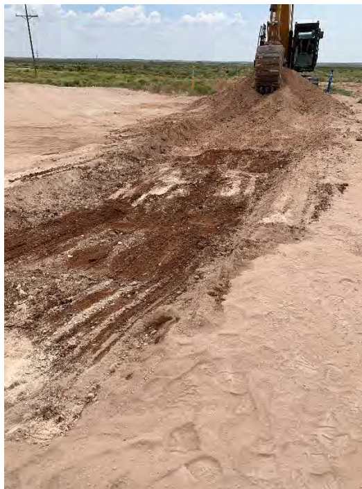
Photo 12: Access Area – scraping surface looking SE
