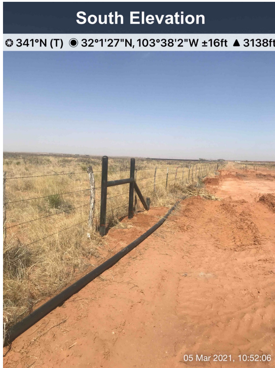
H-Brace constructed to support the fence integrity, March 5, 2021
