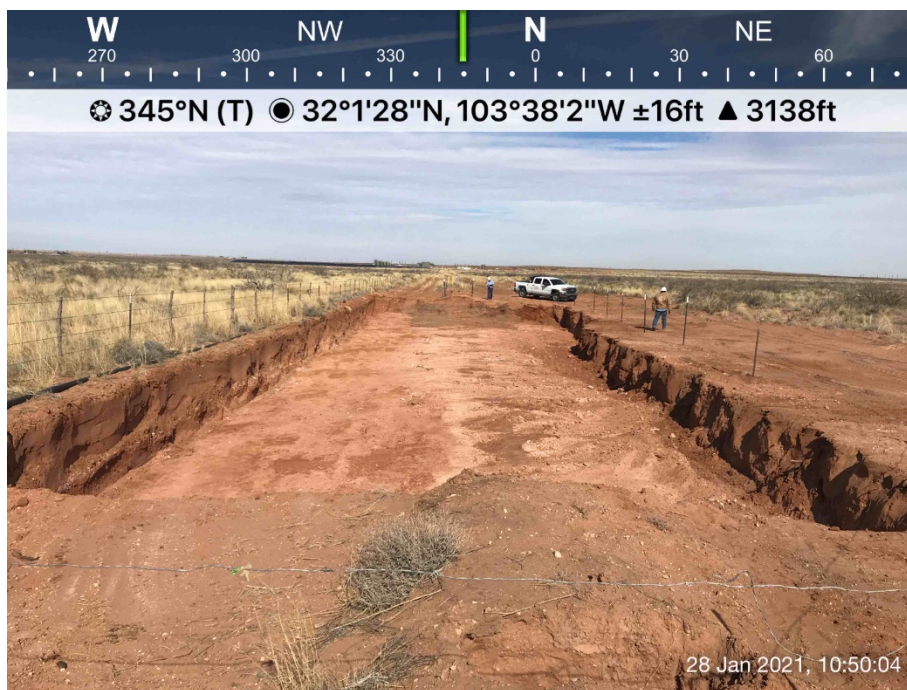
Excavated area to a depth of 4.1 feet bgs, January 28, 2021
