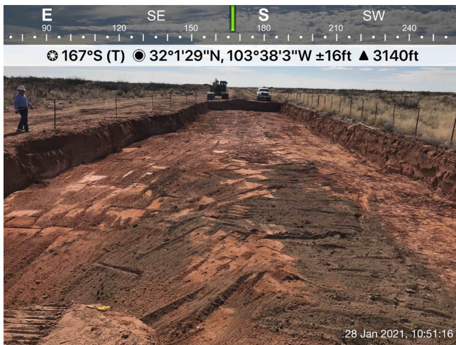
Excavated area to a depth of 4.1 feet bgs, January 28, 2021
