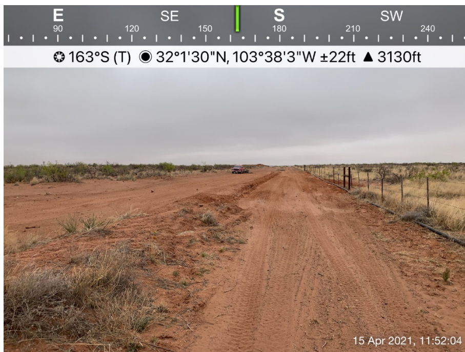
Backfilled and seeded excavation, April 15, 2021
