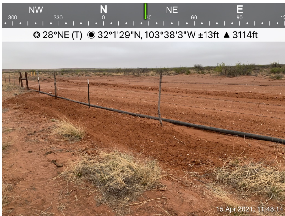
Fence replaced to its original quality, April 15, 2021
