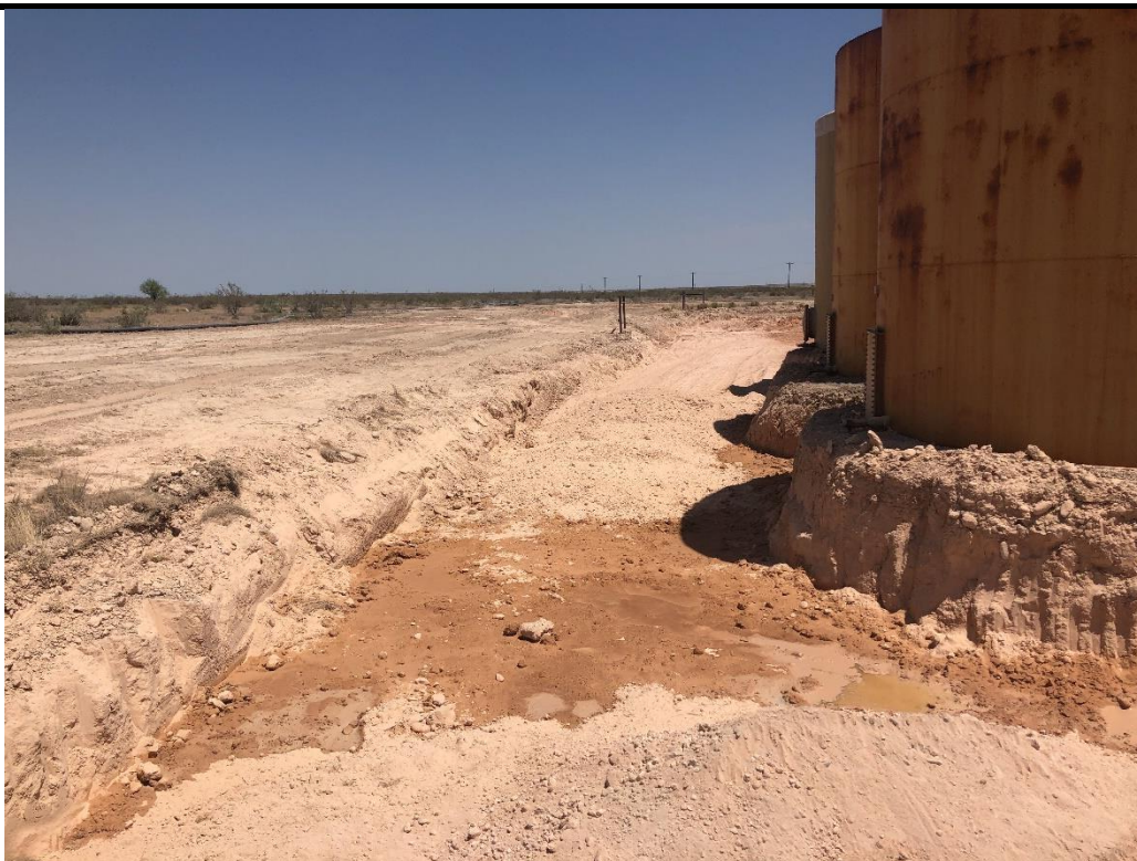
PHOTO 22: View of remediation on west side of tank battery, facing north. 1/28/2020
