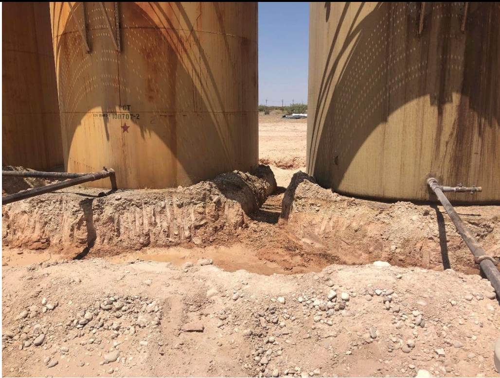
PHOTO 19: View of remediation between tanks, facing west. 1/28/2020
