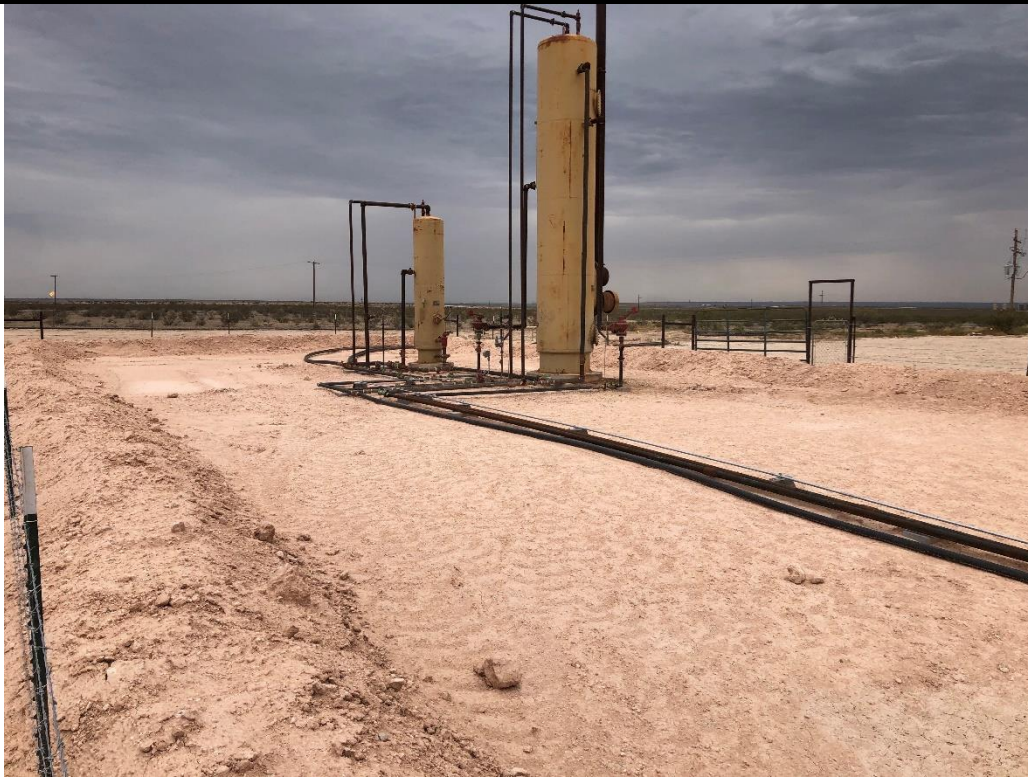
PHOTO 25: View of completed remediation, facing northeast. 8/28/2020
