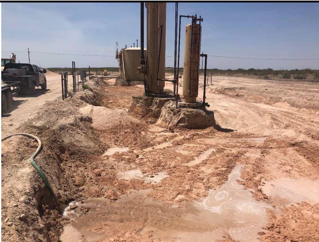
PHOTO 17: View of remediation around heater treaters, facing south. 1/28/2020
