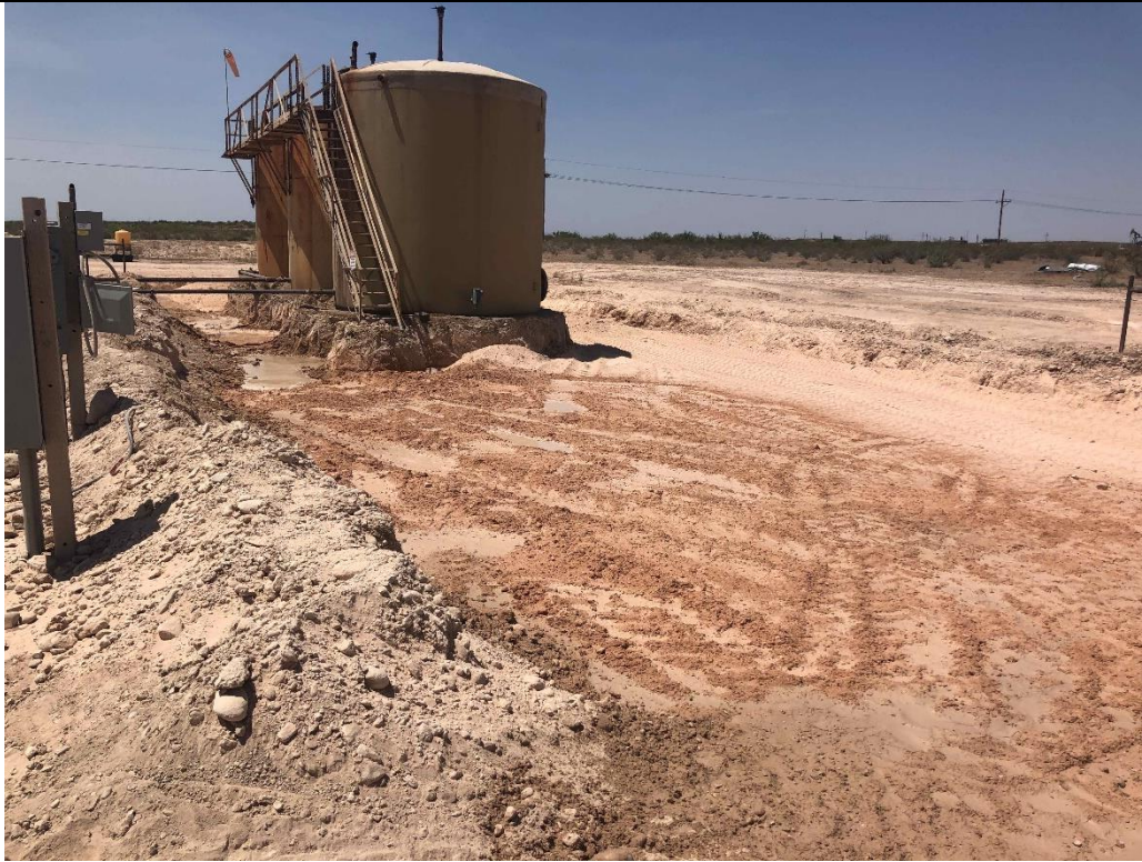
PHOTO 15: View of remediation between the tanks and heater treaters, facing southwest. 1/28/2020
