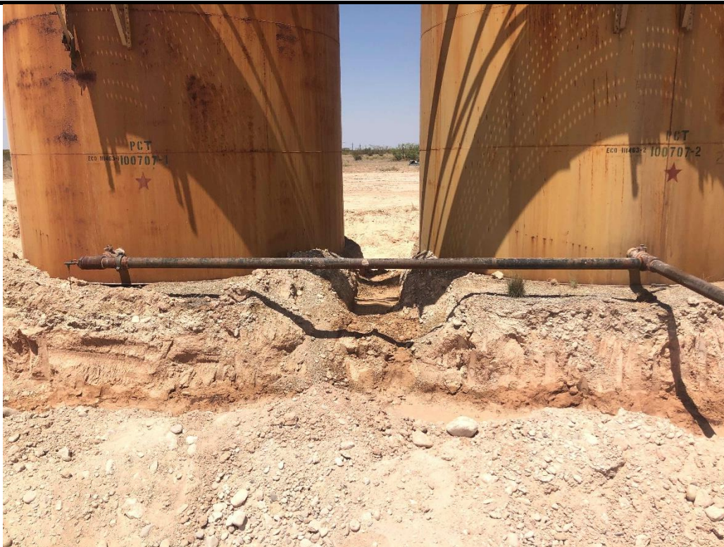
PHOTO 20: View of remediation between tanks, facing west. 1/28/2020
