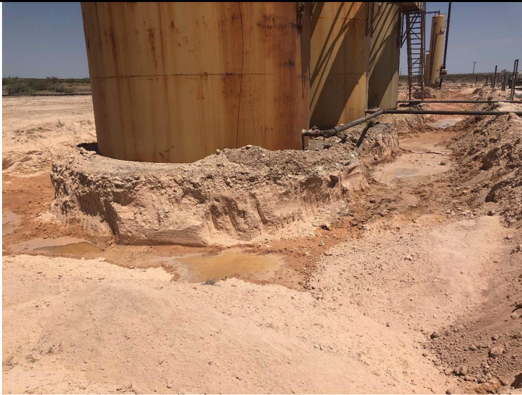
PHOTO 21: View of remediation on east side of tank battery, facing north. 1/28/2020
