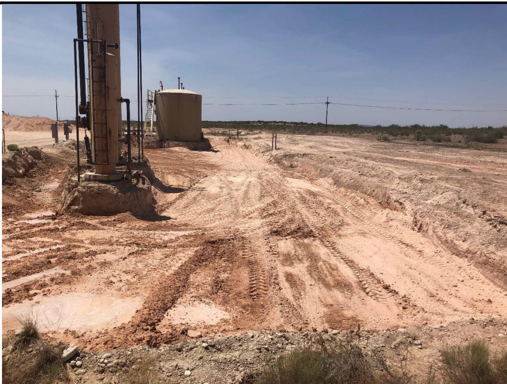
PHOTO 18: View of remediation around heater treaters, facing south. 1/28/2020
