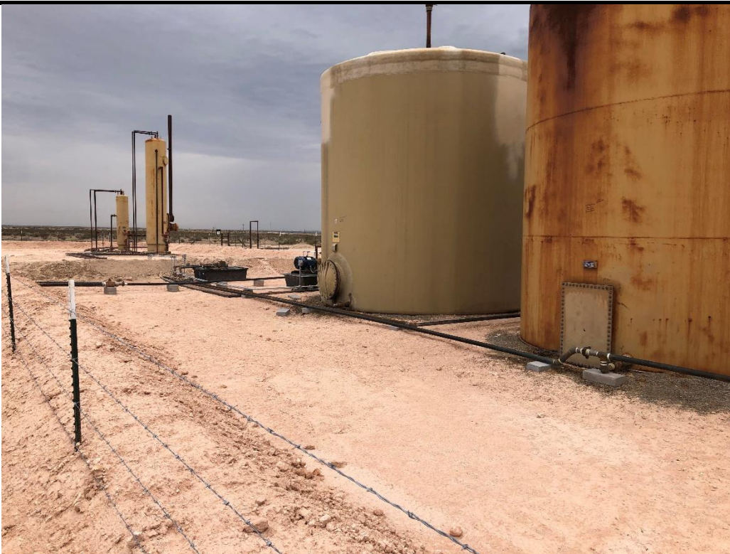
PHOTO 24: View of completed remediation, facing northeast. 8/28/2020
