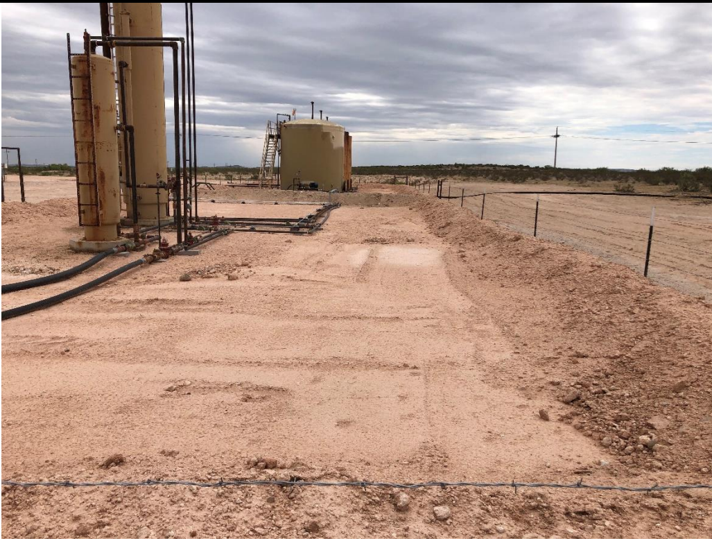
PHOTO 23: View of completed remediation, facing south. 8/28/2020
