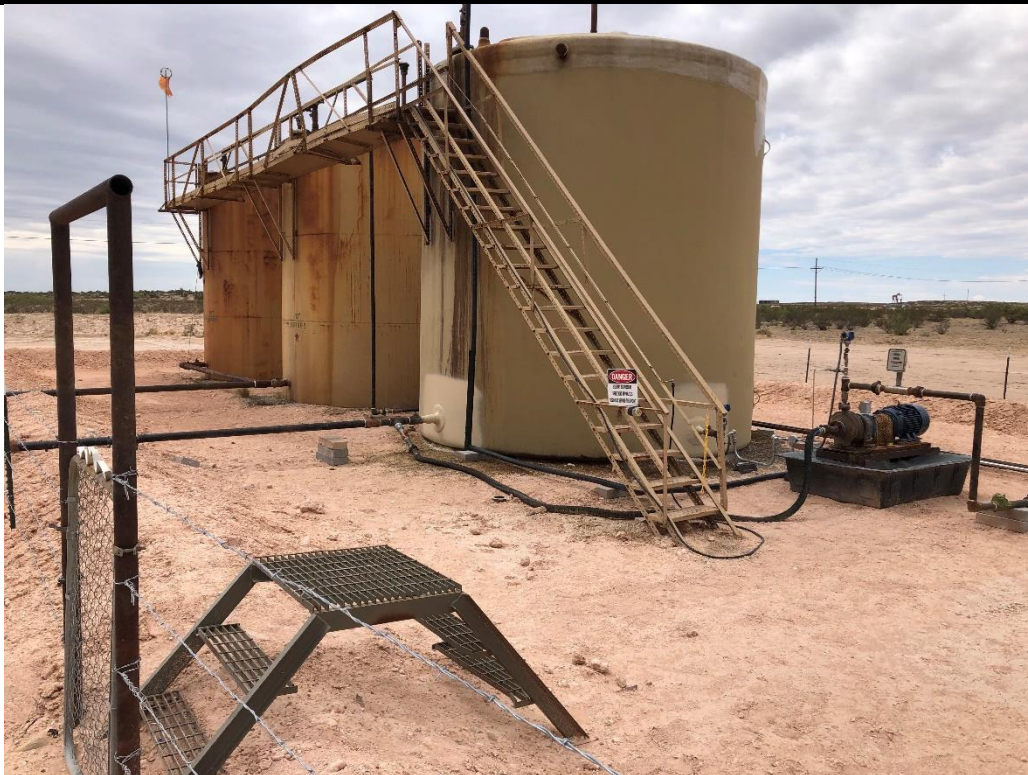
PHOTO 26: View of completed remediation, facing southwest. 8/28/2020
