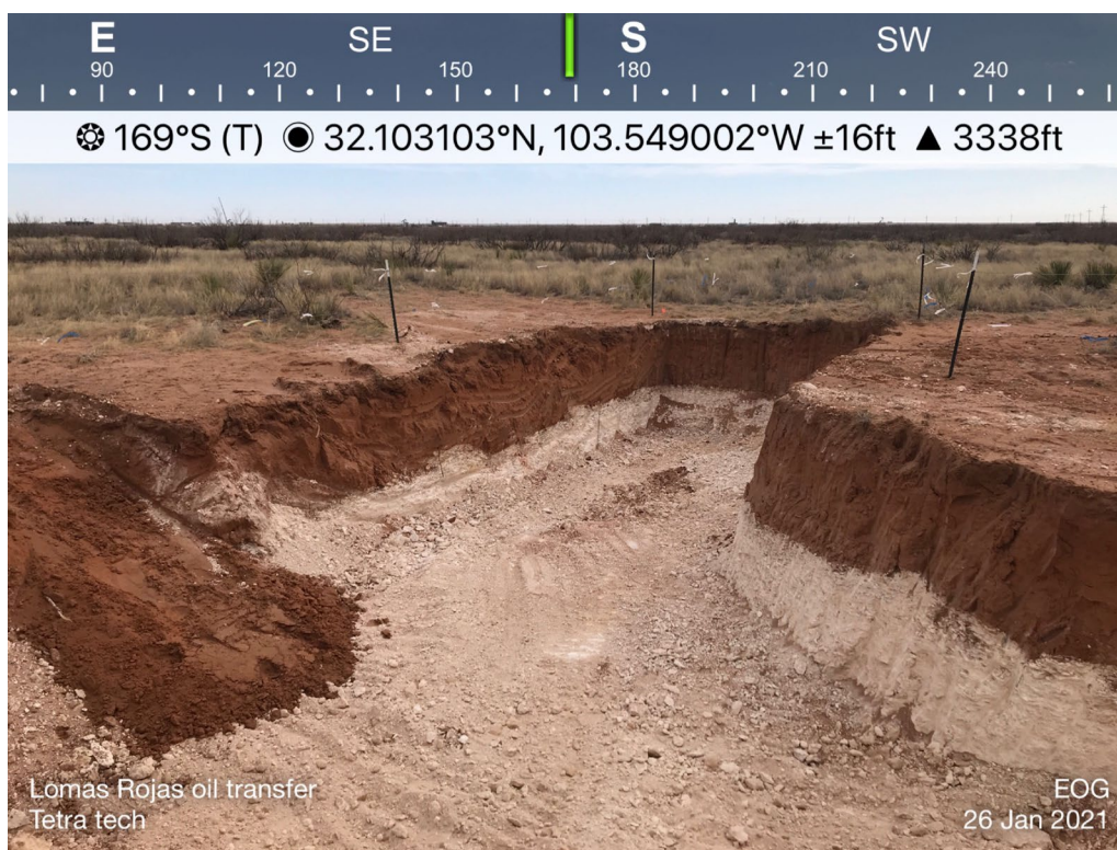
View of Remediation Activities– View South
