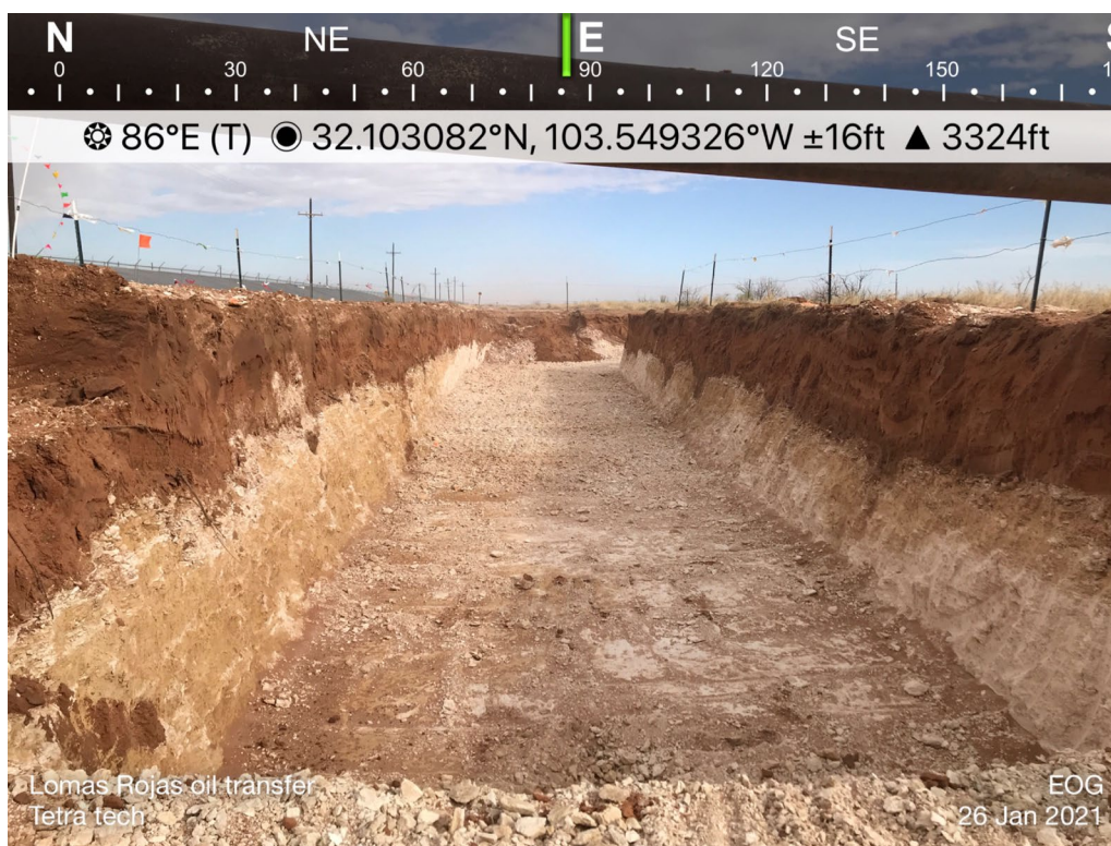
View of Remediation Activities – View East
