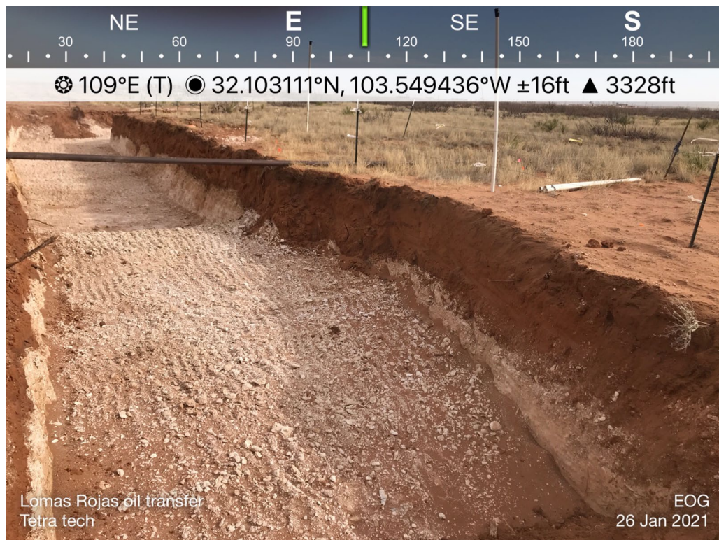
View of Remediation Activities – View East
