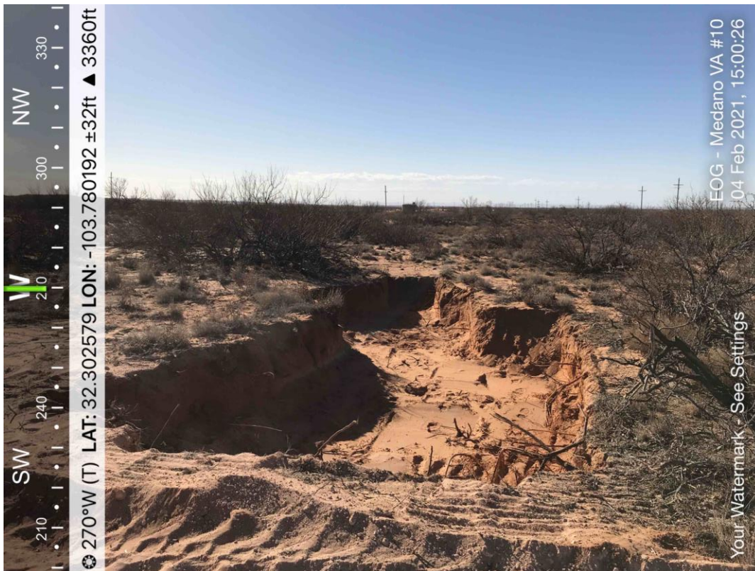
View of Remediation Activities – View West
