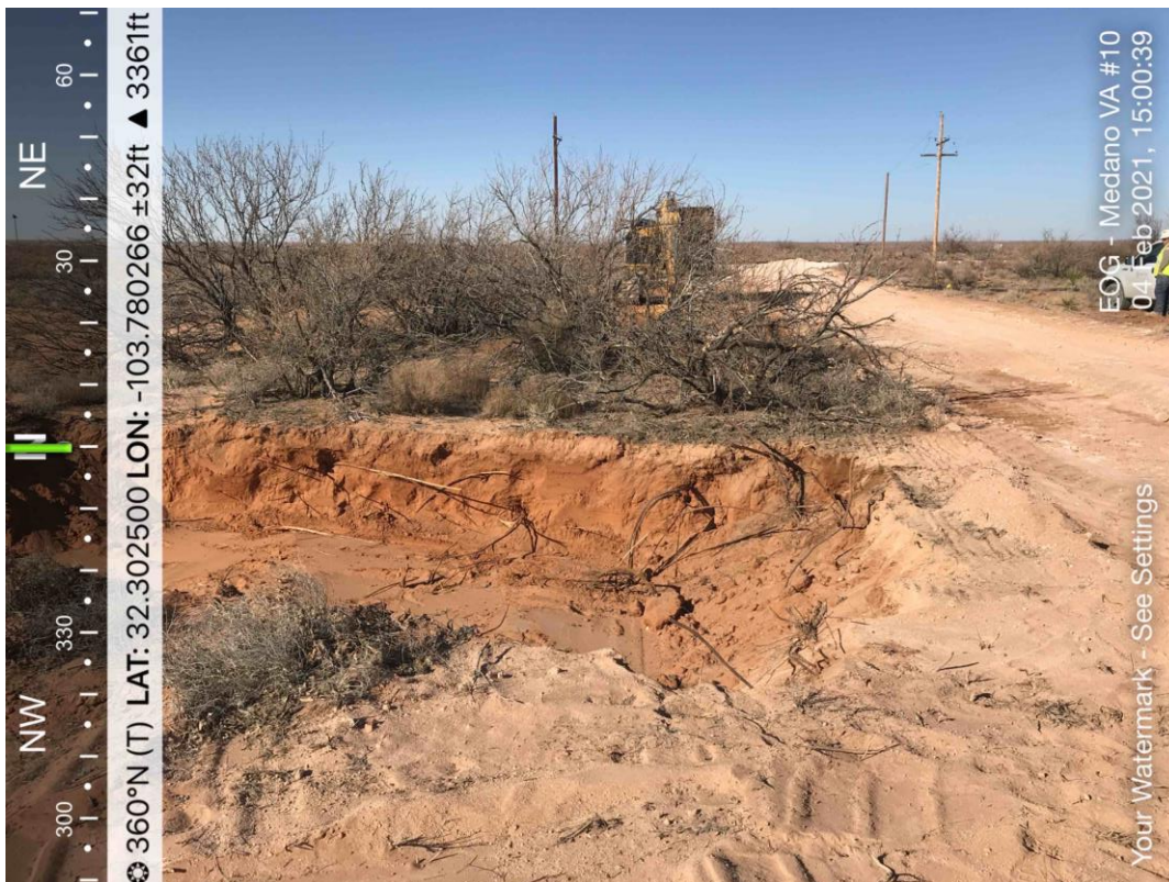
View of Remediation Activities – View North
