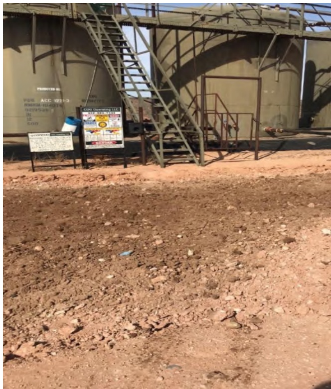
Excavated area of AH-1 and AH-2
