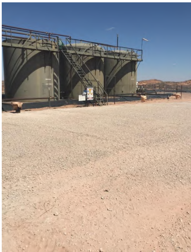
Backfilled area of AH-1 and AH-2
