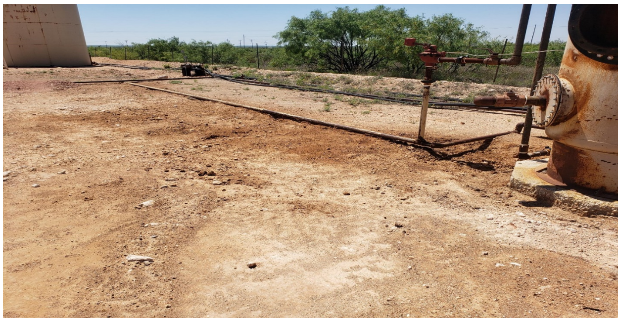
REMOVAL OF 0.5" - 1' AROUND HEATER AND LINE GOING TO BATTERY
