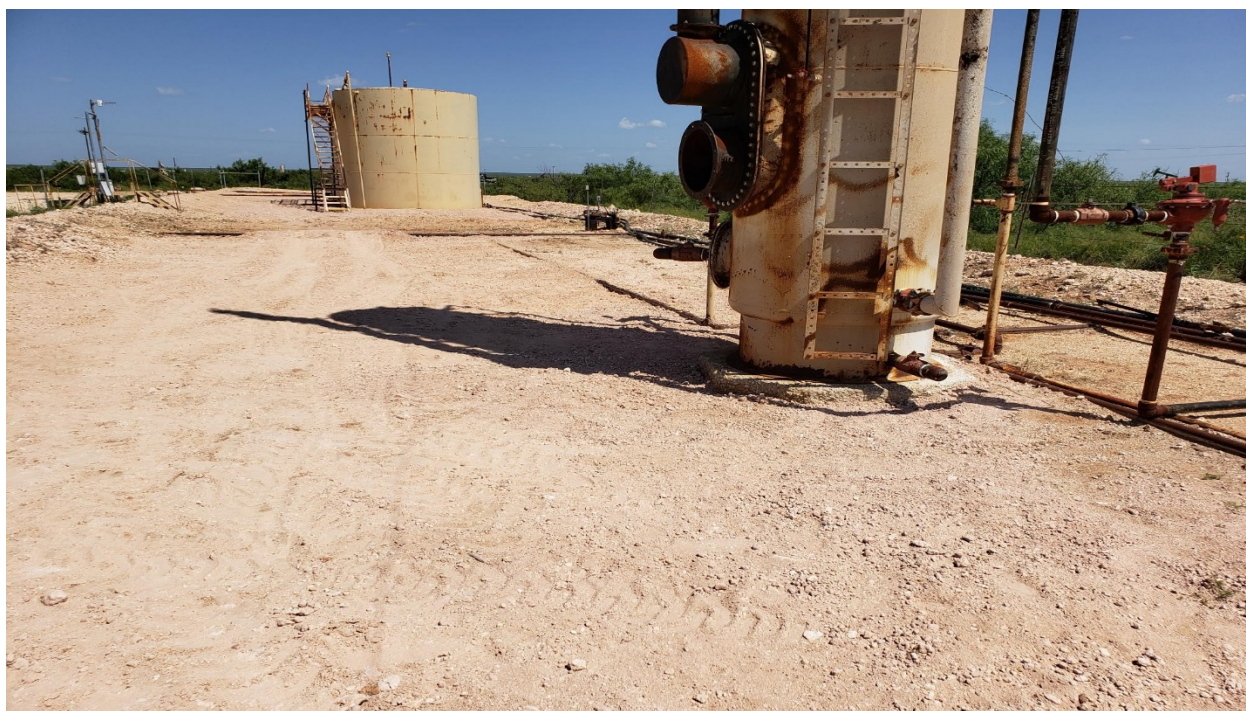
BACKFILL OF CALICHE AROUND HEATER AND LINE GOING TO TANKS
