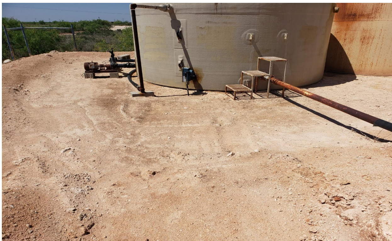
REMOVAL OF 0.3"-0.5" OF CALICHE AROUND TANKS WITH MACHINERY AND HAND EQUIPMENT
