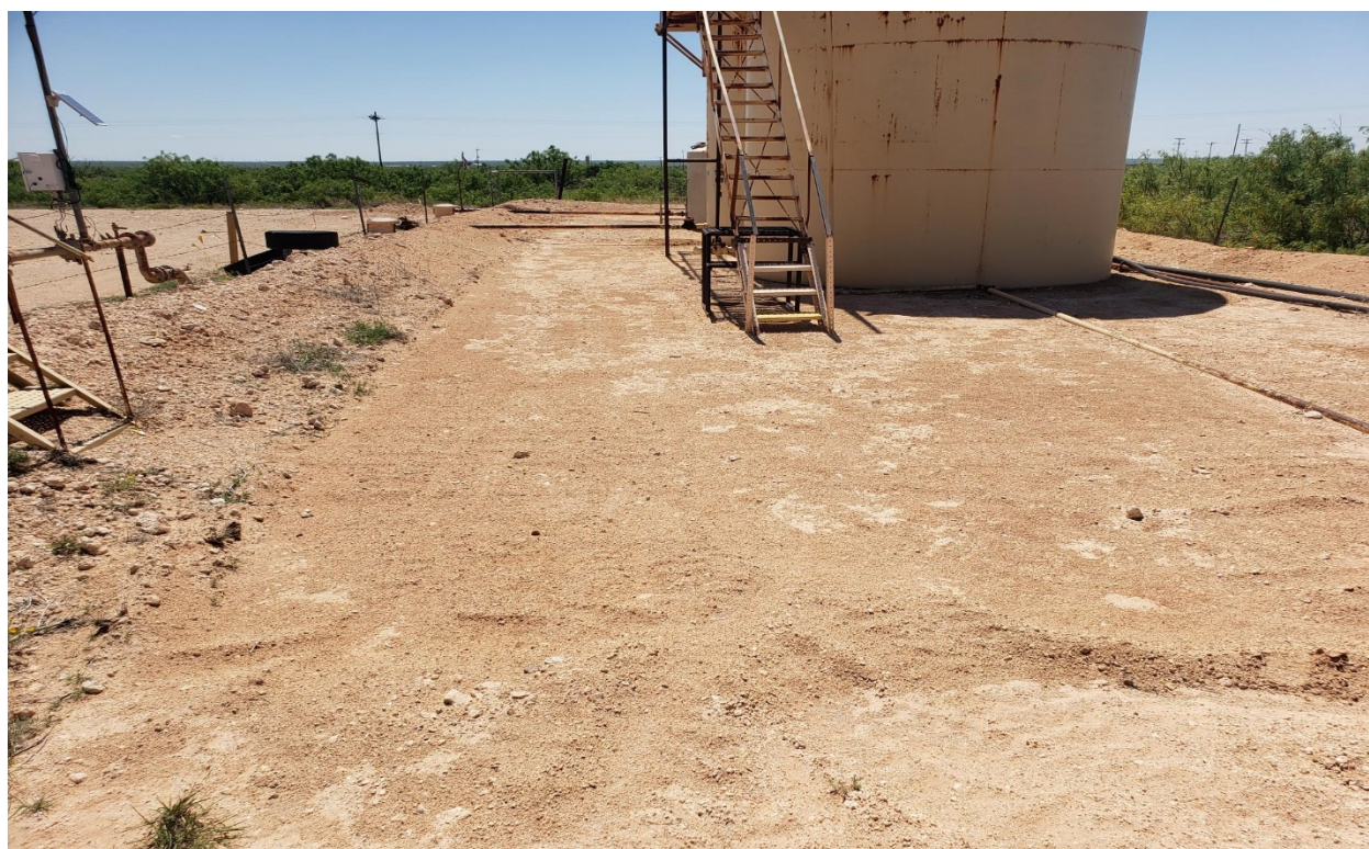
REMOVAL OF 0.3"-0.5" CALICHE AROUND TANKS
