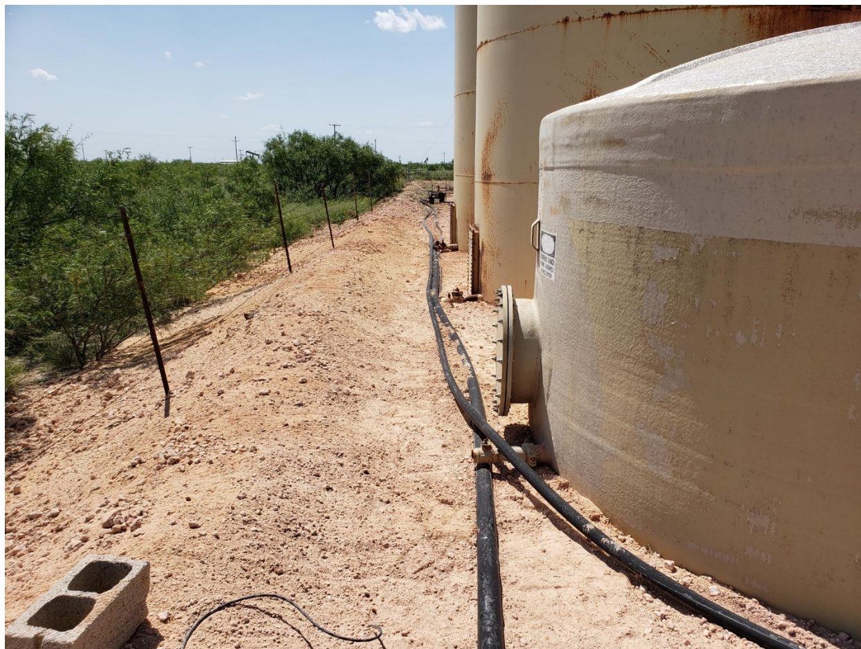
BACKFILL AROUND BACK OF TANKS AND BETWEEN TANKS
