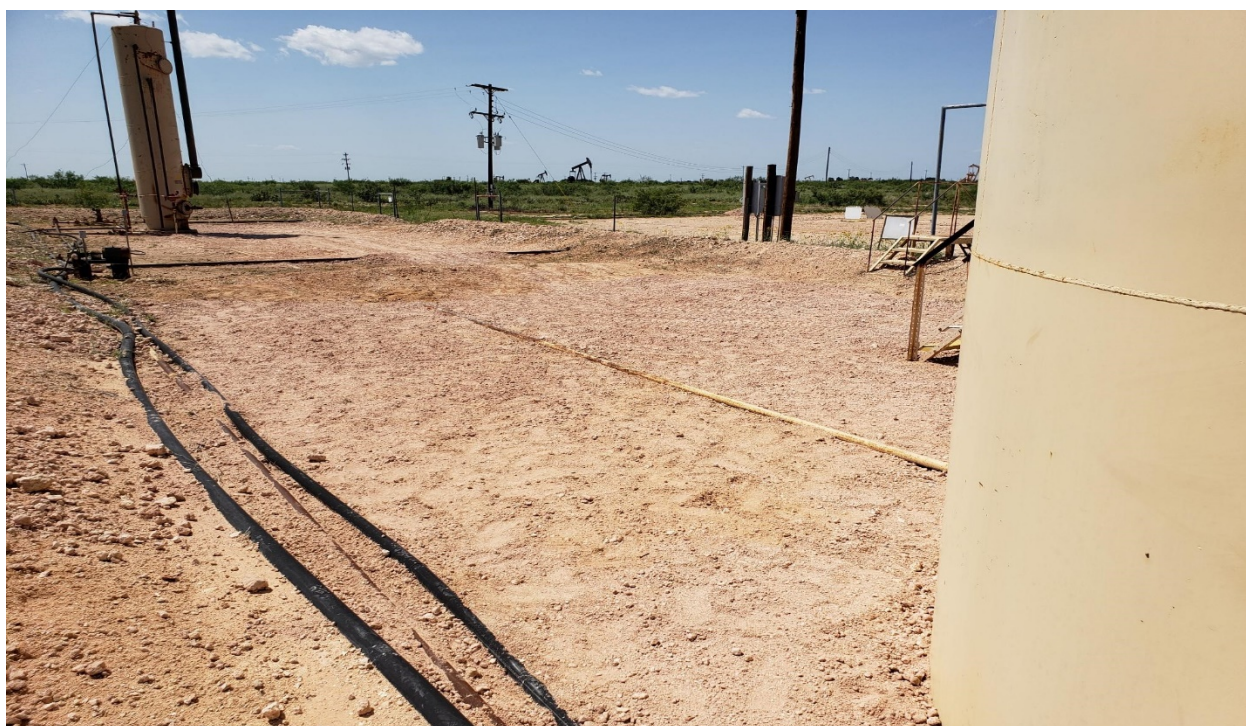
BACKFILL OF CALICHE AROUND TANKS AND FRONT OF HEATER
