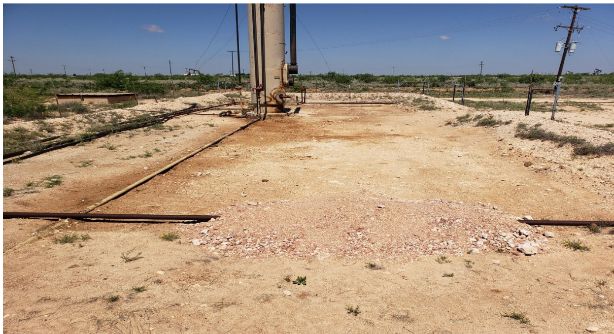
REMOVED 0.5"-1' OF CALICHE DOWN TO NON IMPACTED SAND AROUND HEATER AND LINES
