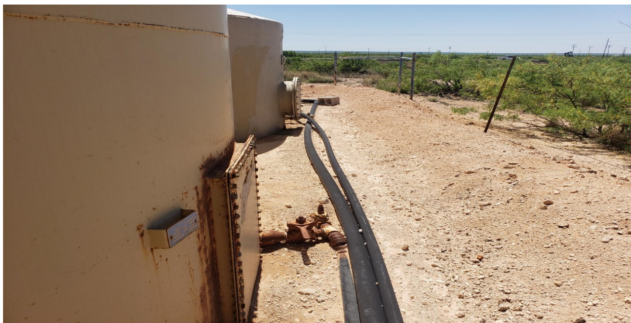
REMOVAL OF 0.3"-0.5" OF CALICHE AROUND TANKS
