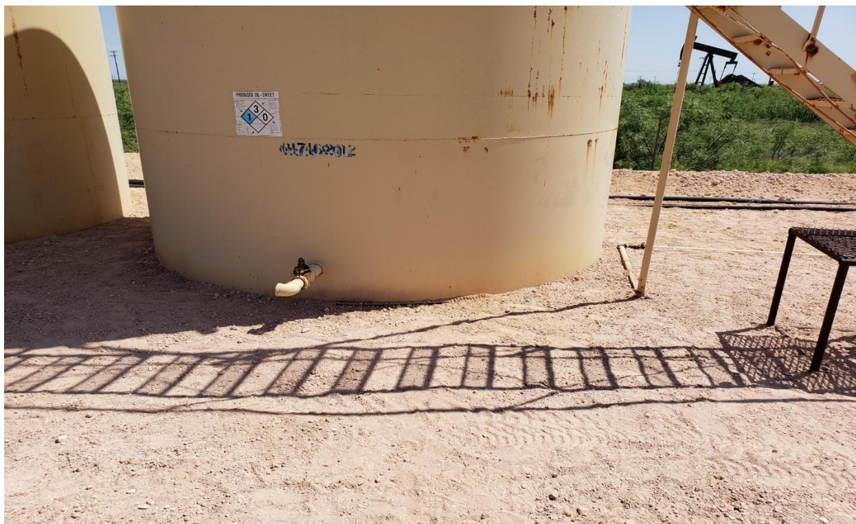
BACKFILL OF CALICHE AROUND TANKS
