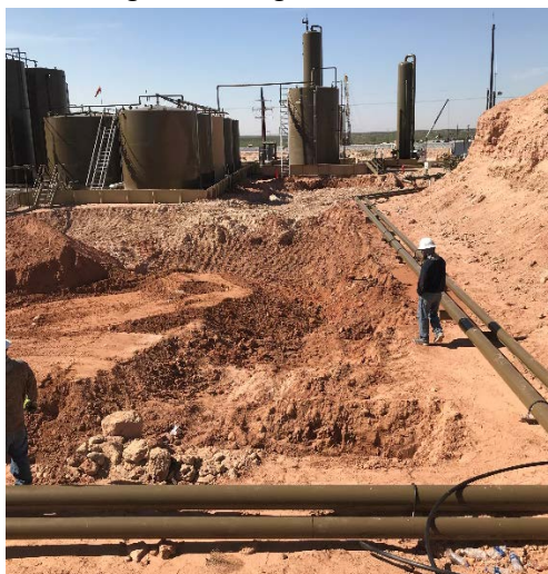
Photograph 5: South facing view during excavation activities.
