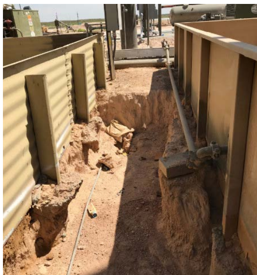
Photograph 3: View of open excavation between containments.
