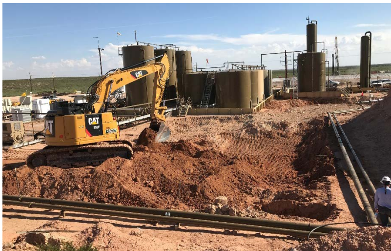
Photograph 4: South facing view during excavation activities.
