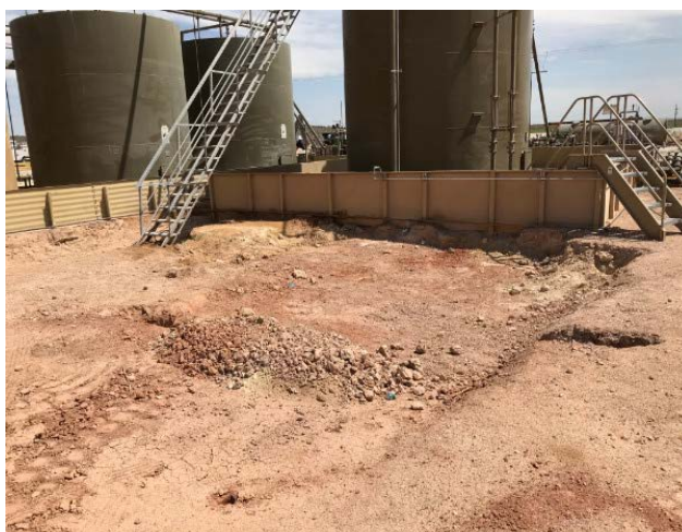
Photograph 2: Southeast facing view during excavation activities.
