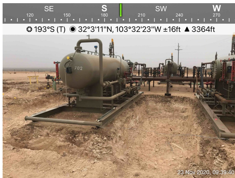
View of Remediation Activities – View South
