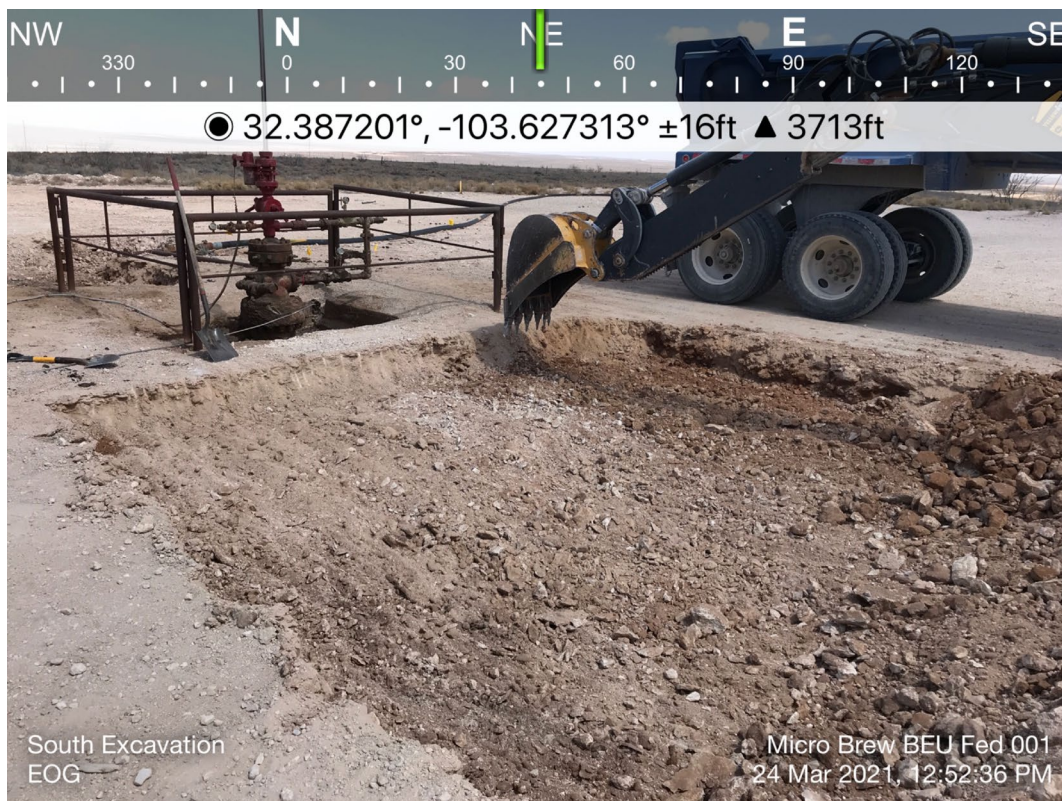
View of Remediation Activities– View Northeast
