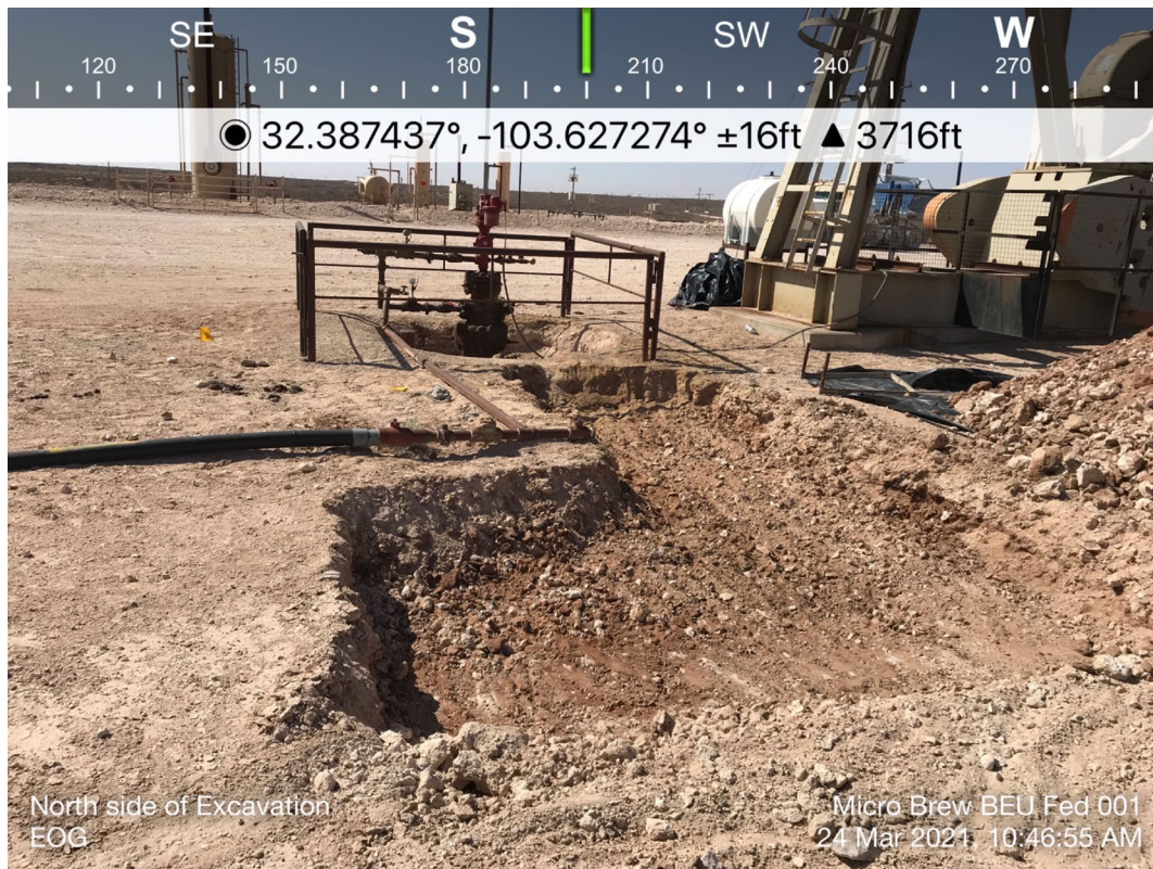
View of Remediation Activities – View South
