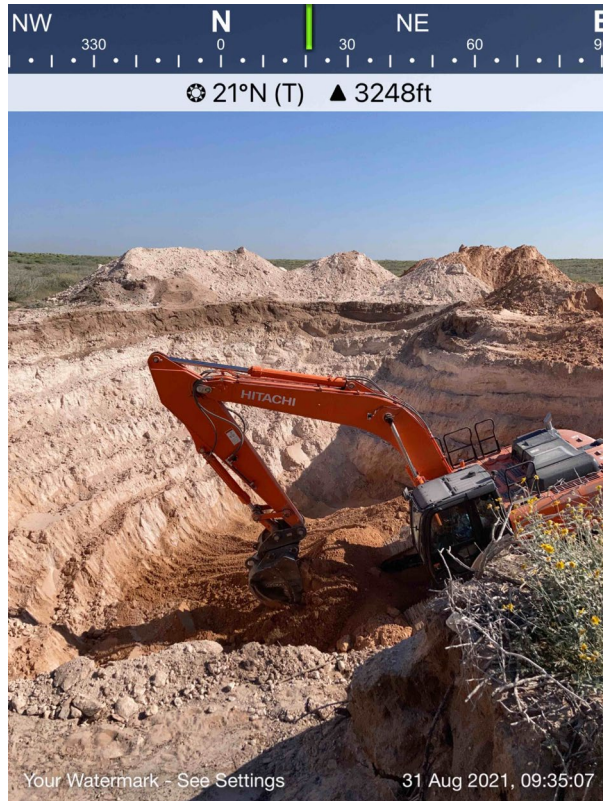
View of Remediation Activities – View Northeast
