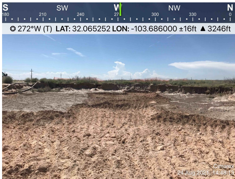
View of Remediation Activities – View West
