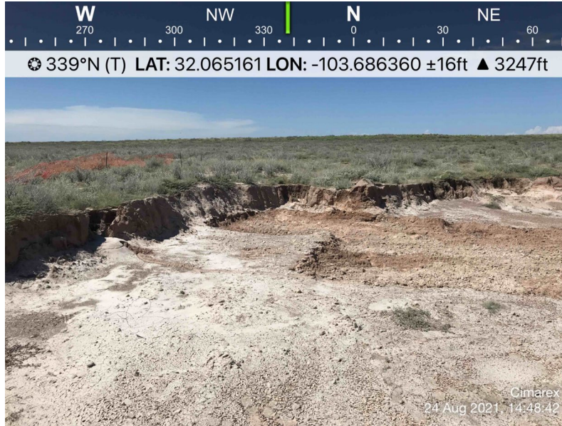
View of Remediation Activities – View Northwest
