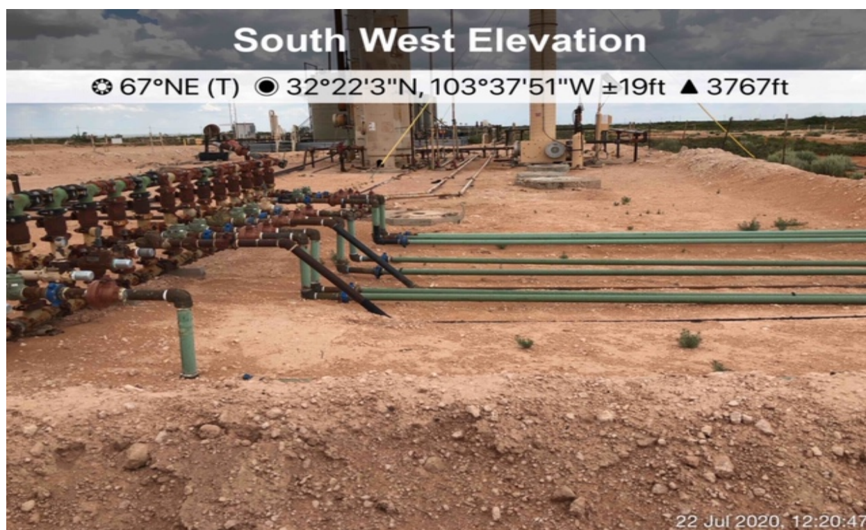
Remediated Source Area at Manifold. Rebuilt Berms in Foreground Looking Northeast
