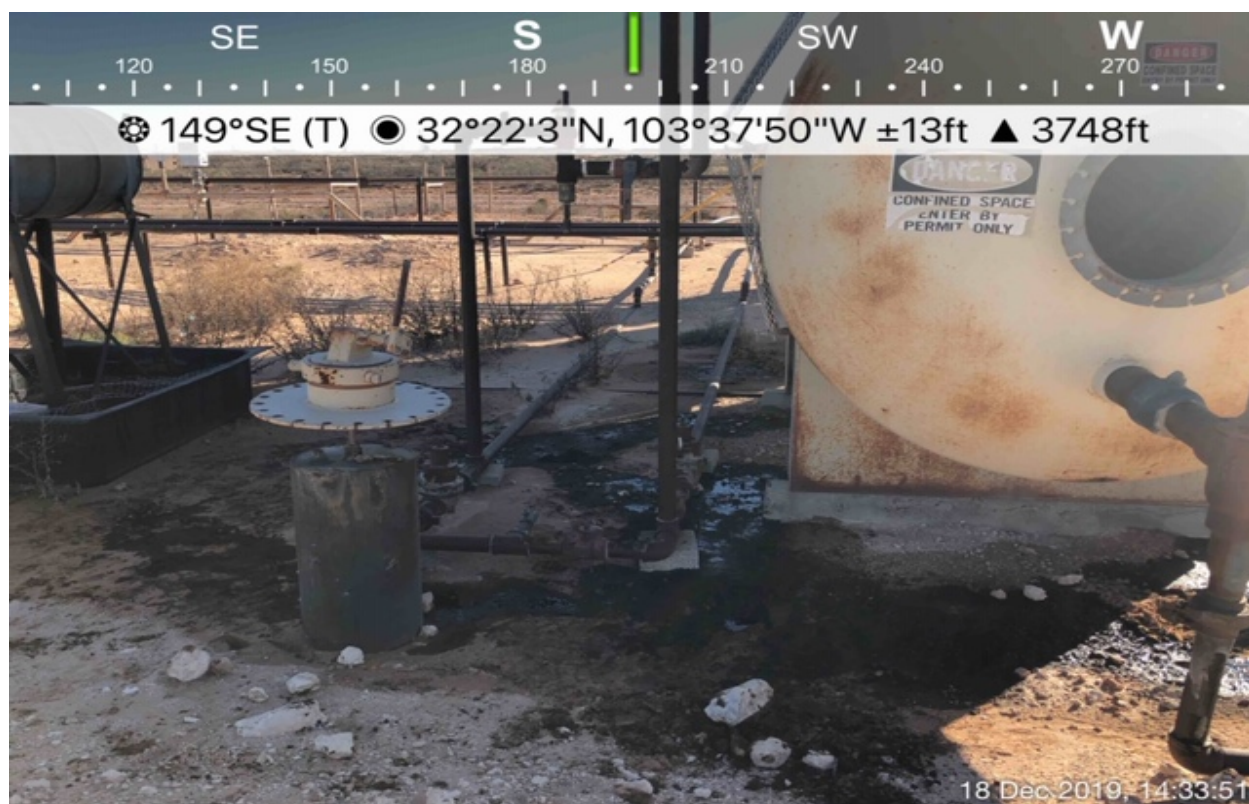
Standing Oil and Produced Water Staining Near East Terminus of the Release
