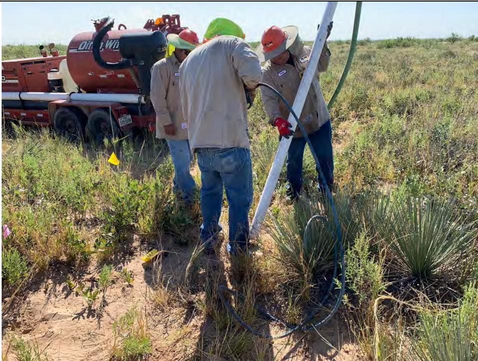
Photo 5: View facing southeast of hydro-excavation activities of underground gathering line by Talon LPE in order to confirm location of line prior to nearby drilling activities at SB-29.
