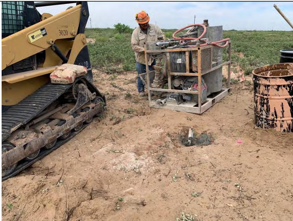
Photo 2: View looking northwest of the downhole grouting activities of MW-05 by Talon LPE. The monitoring well was advanced approximately 85 feet northwest of the release point.
