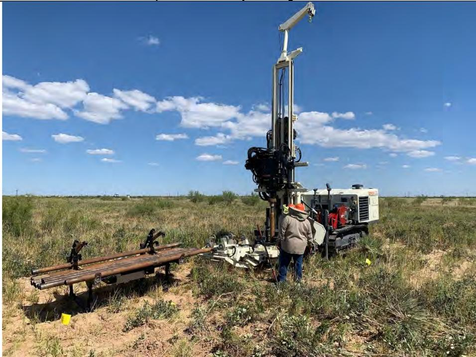
Photo 6: View facing northeast of Talon LPE subsurface soil boring advancement at SB-29. Soil boring is located approximately 90 feet east of release point and 6 feet north of underground gathering line.
