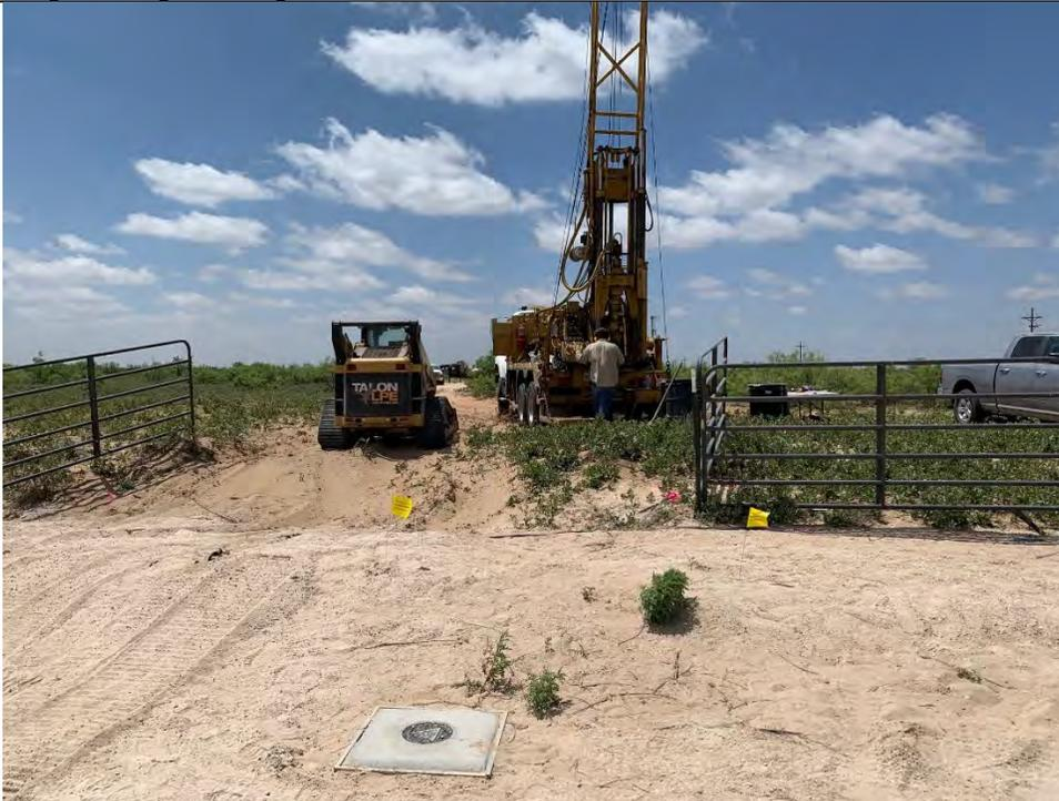
Photo 4: View facing south of Talon LPE subsurface soil boring advancement at SB-26. The yellow flags inside the fenced area mark the location of the WTX to EMSU Battery to Byrd Pump Segment gathering line.
