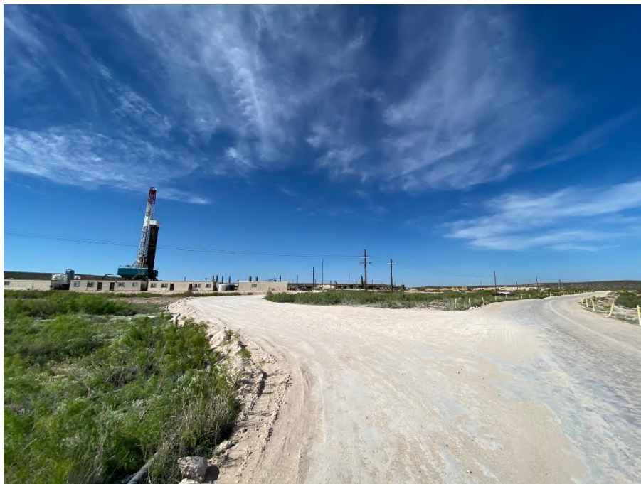
Photograph 5: North facing view of new lease road constructed over the north side release area.
