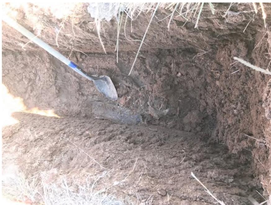
Photograph 4: View of the installed liner in the excavation north of the road.
