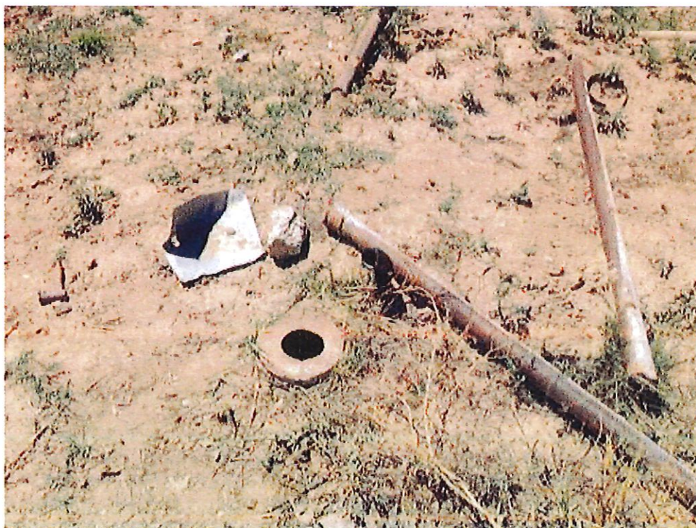
Top of open well at ground surface
