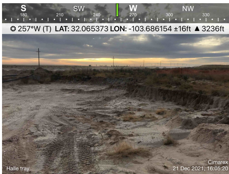
View of Remediation Activities – View West
