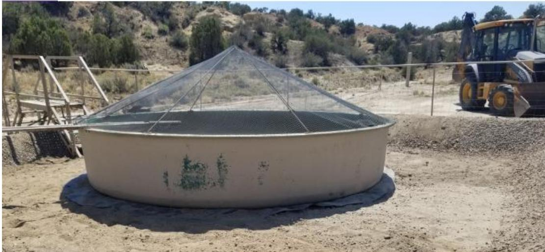
An Above Grade Tank (AGT) has been placed in the area where the BGT was previously located. The ground has been leveled up to match the contour of the site and a berm built around the AGT.
