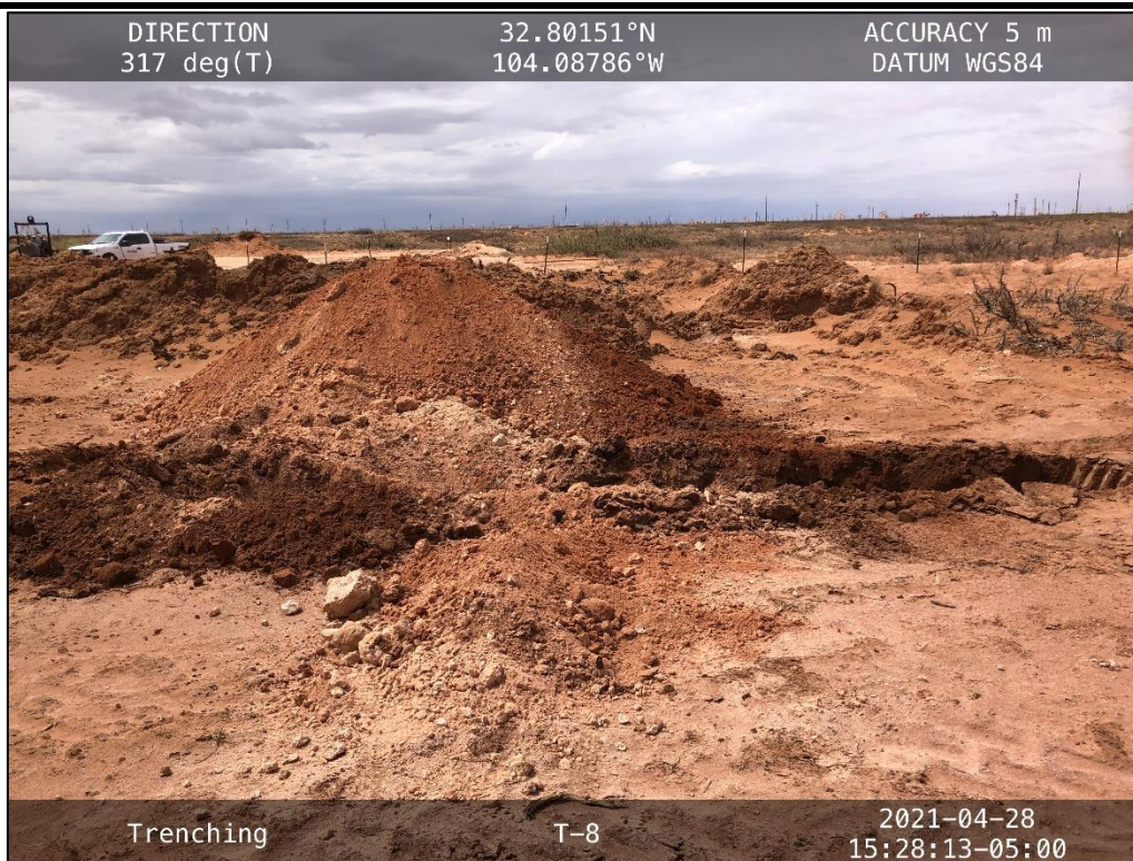
PHOTO 16: View of trenching.
