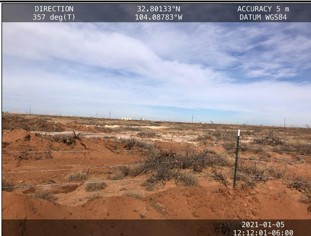
PHOTO 8: View of Seep impacts.
