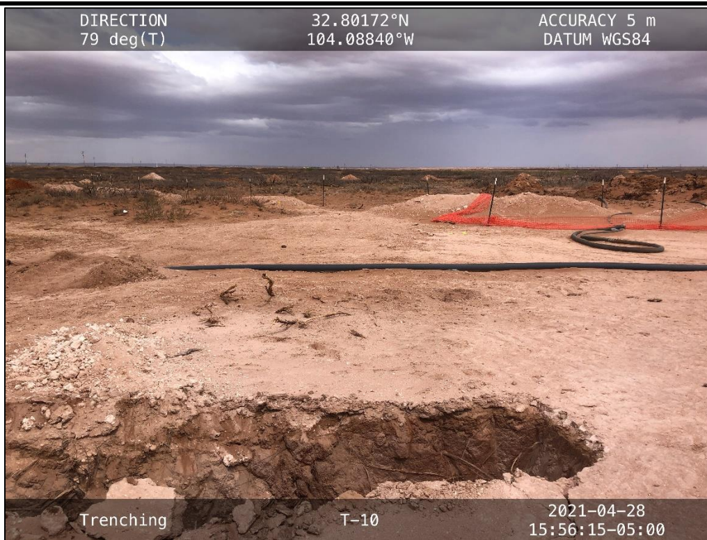
PHOTO 17: View of trenching.
