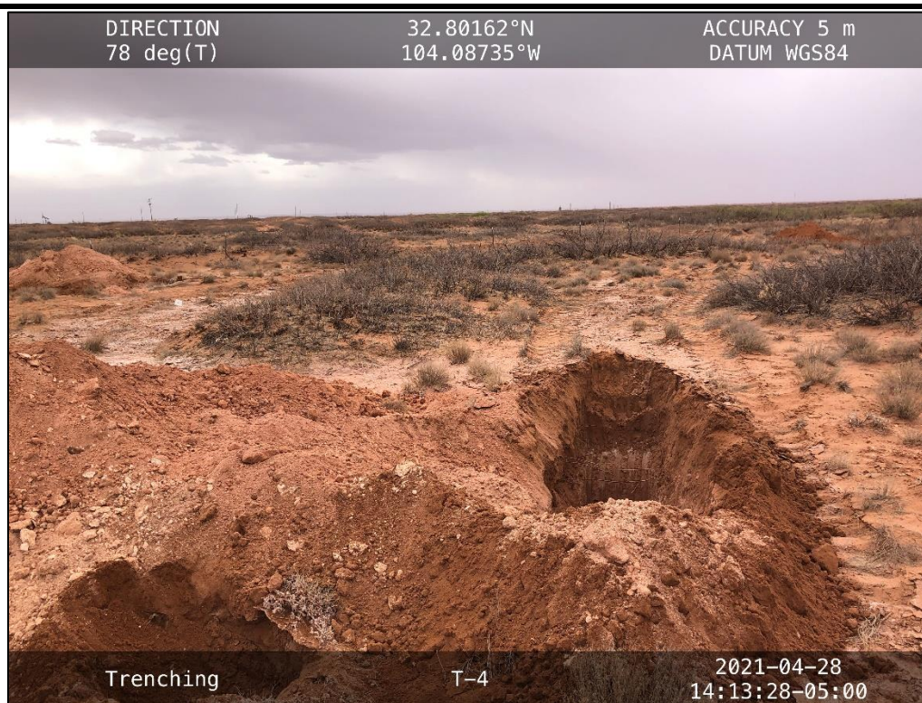
PHOTO 15: View of trenching.
