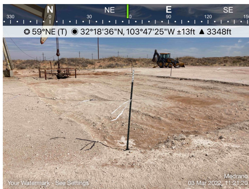
View of Remediation Activities – View Northeast
