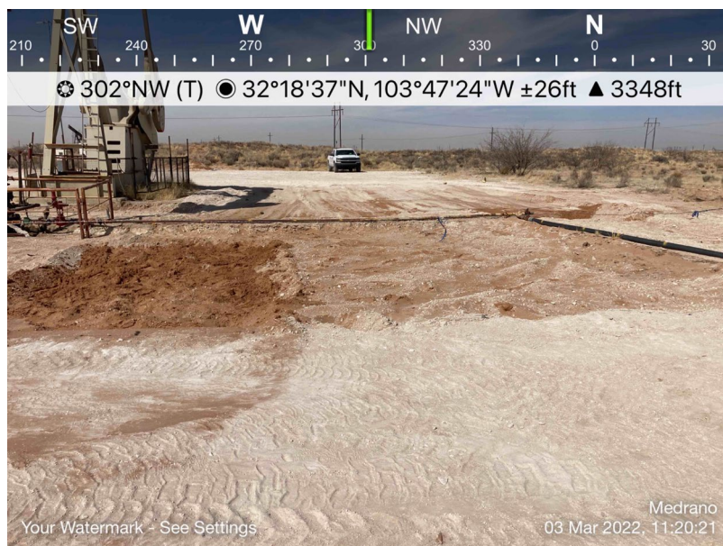
View of Remediation Activities – View Northwest
