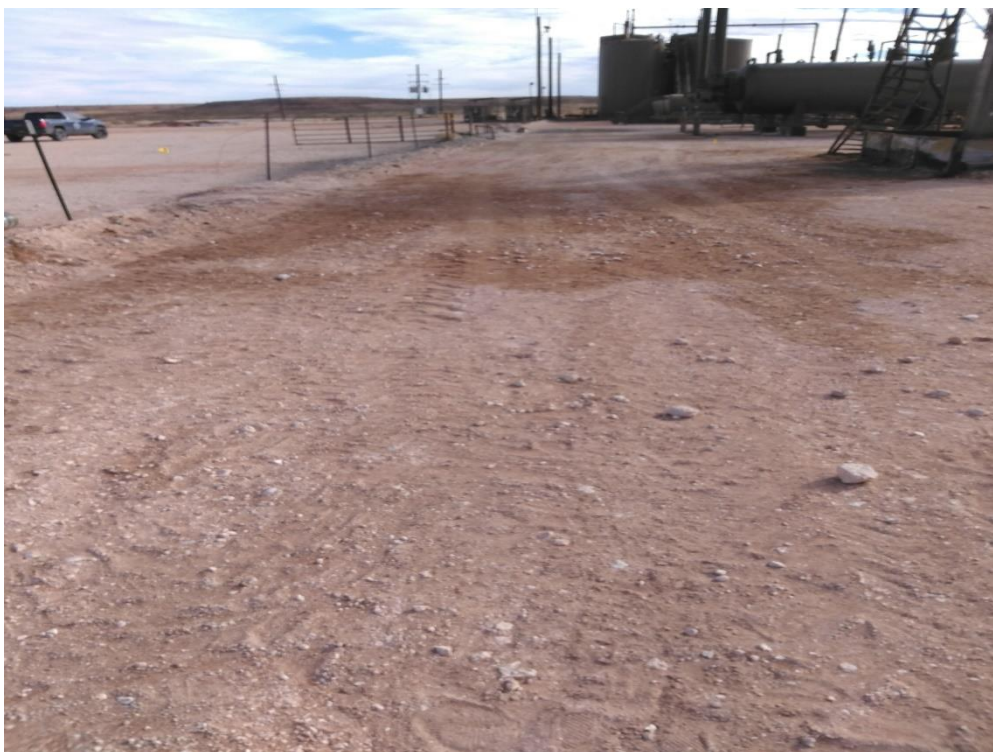
Photo 4: View of soil staining along the facility's northern containment berm facing east
