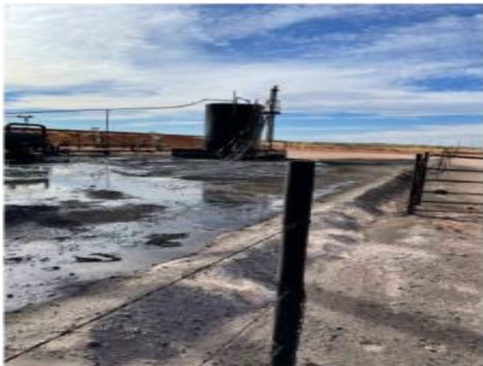
Photo 1: View of fluid covering the ground surface facing west-southwest
