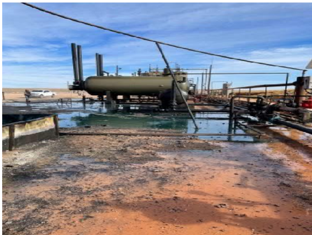
Photo 2: View of fluid covering the ground surface facing east
