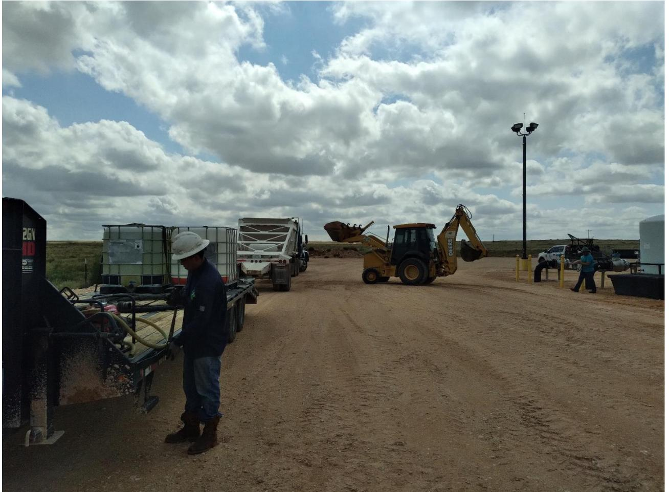
**Figure 7:** Removal of Top Layer of Contaminated Soil Using Backhoe and belly-dump trucks
