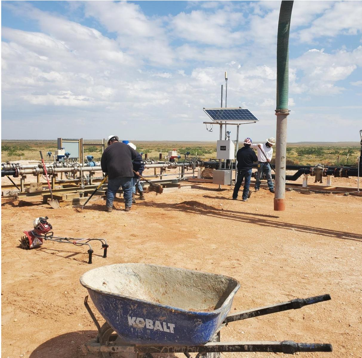
**Figure 4:** Removal of Top Layer of Contaminated Soil Near Pipes of Location Cheddar RP SWD
