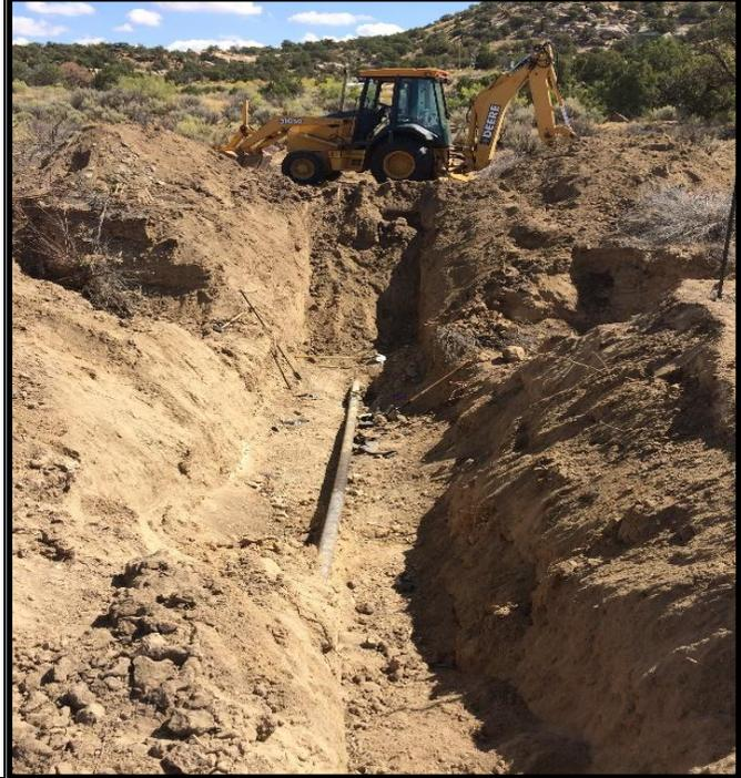
Figure 2. Excavation activity following the removal of the pipeline.
