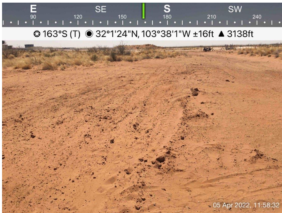
Hydrovac-2 backfilled and seeded excavation viewing south
