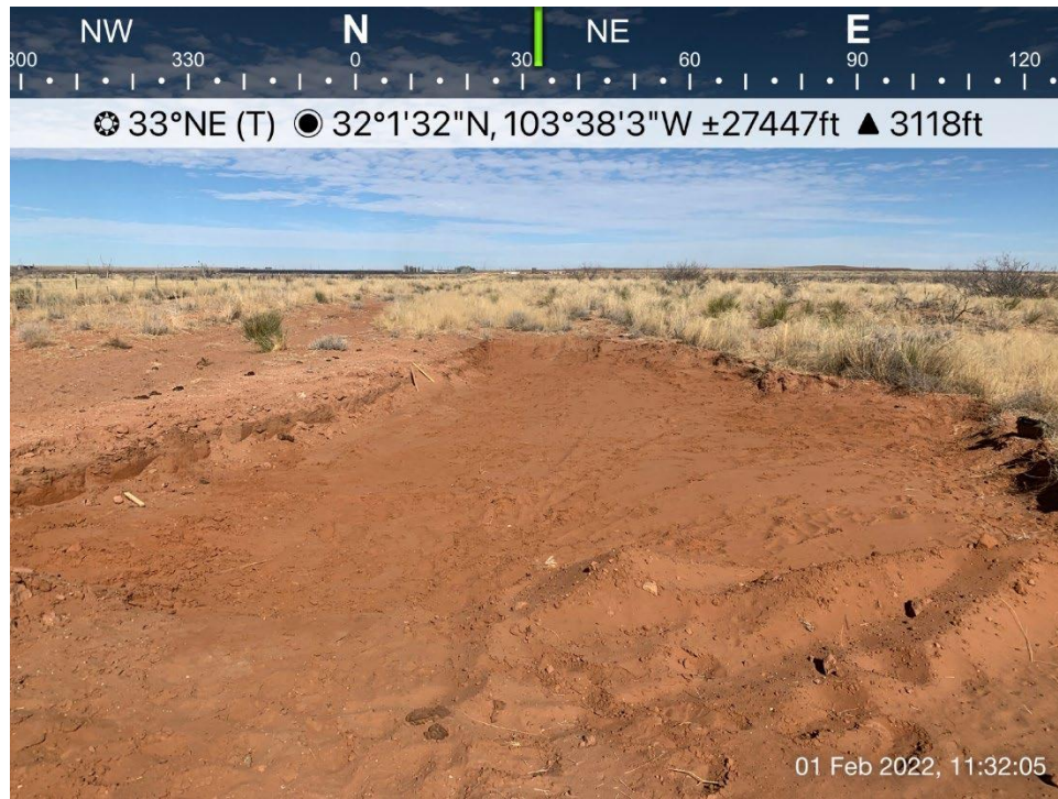
Hydrovac-1 excavated soil viewing northeast
