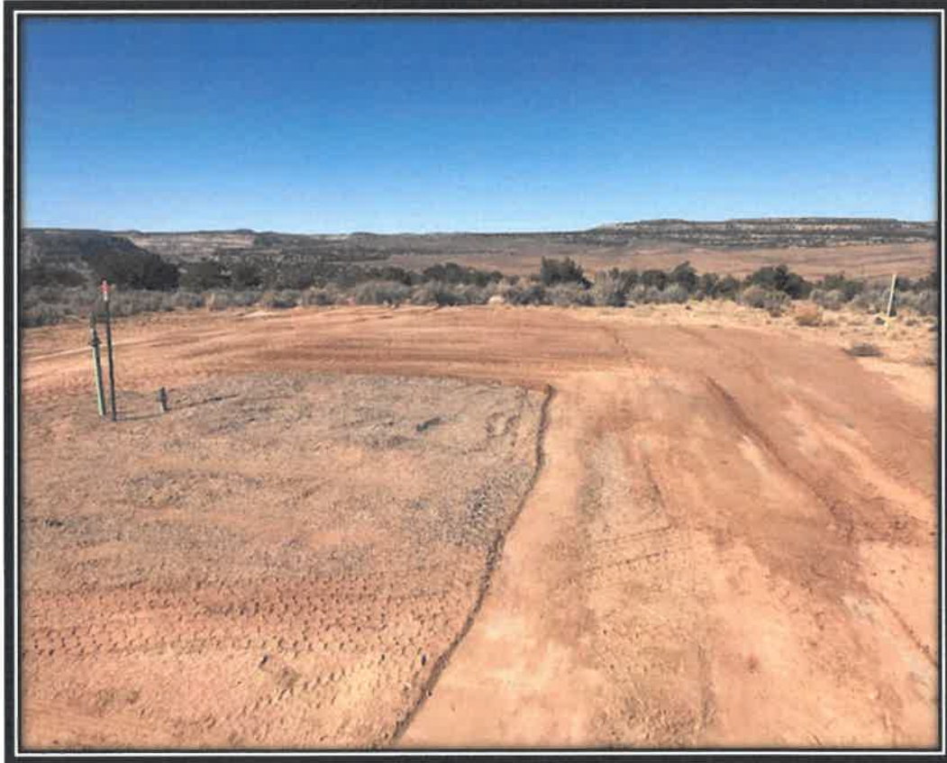
Photo: Area Backfilled
