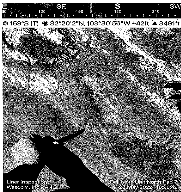
Liner Bubble ( Near Tank 1196)
