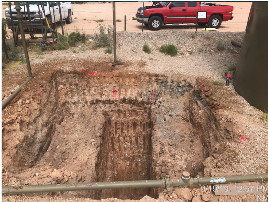
View North – Excavated Area
