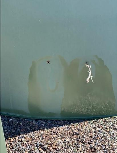
A close-up photograph of the green cylindrical storage tank. Two distinct bullet holes are visible in the metal surface of the tank. The tank is situated on a gravel pad.                                                                                                                                  |
