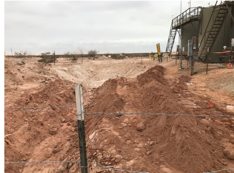
Photograph 2: View of pad and excavation – looking west
