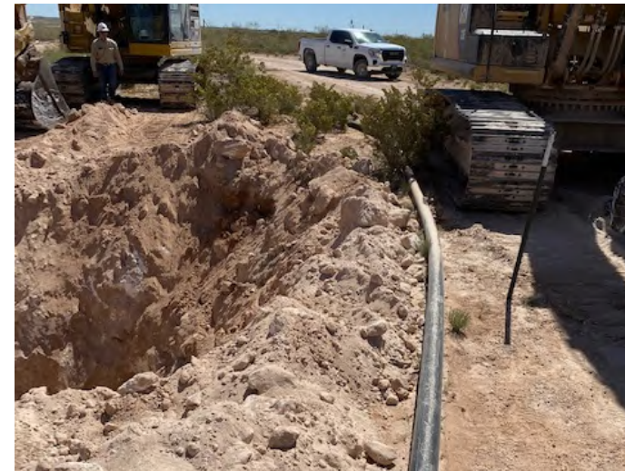
Photograph 4: View of open excavation – looking east.
