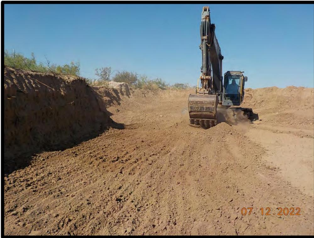
**PHOTOGRAPH NO. 3 – A view of over-excavation activities in the “EX-2” sample area on July 12, 2022. The view is towards the southwest.**
