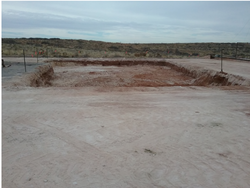
View North – Excavation Area
