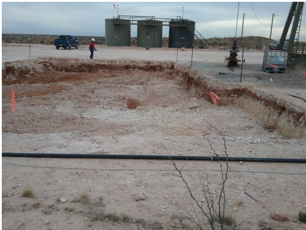
View South – Excavation Area
