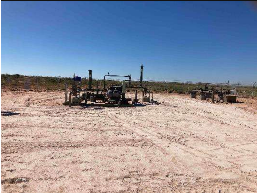
PHOTO 12: View of the remediated area facing south. 9/20/22
