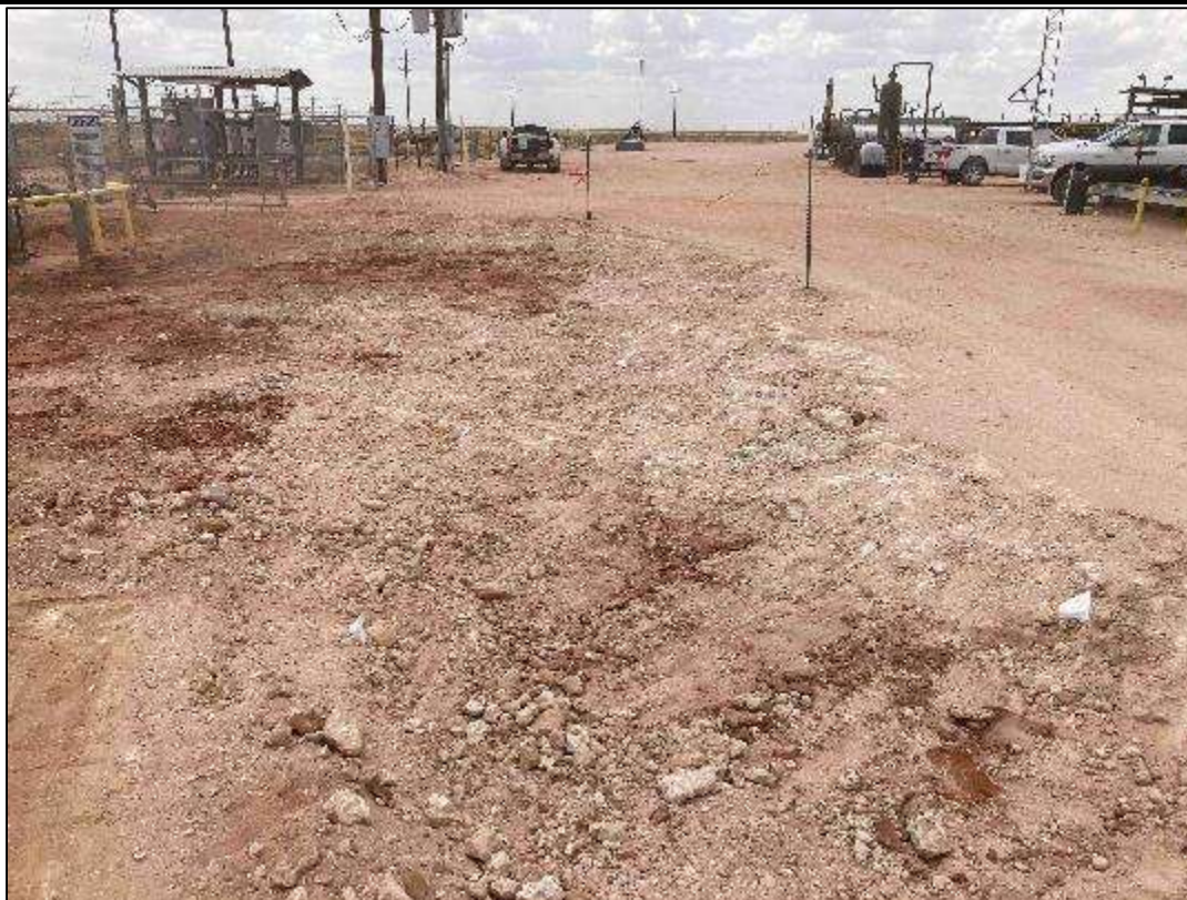
PHOTO 5: View of the excavated area facing west. 8/11/22
