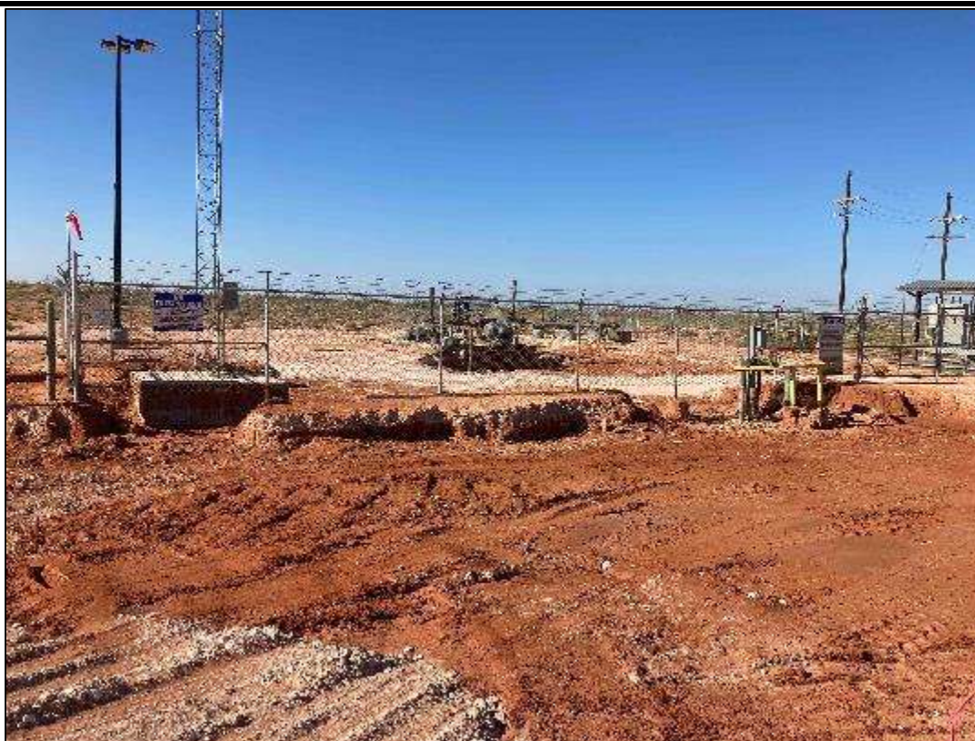
PHOTO 10: View of the excavated area facing south. 8/29/22
