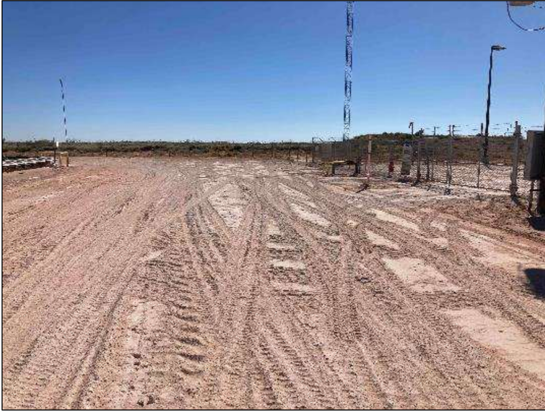
PHOTO 11: View of the remediated area facing east. 9/20/22
