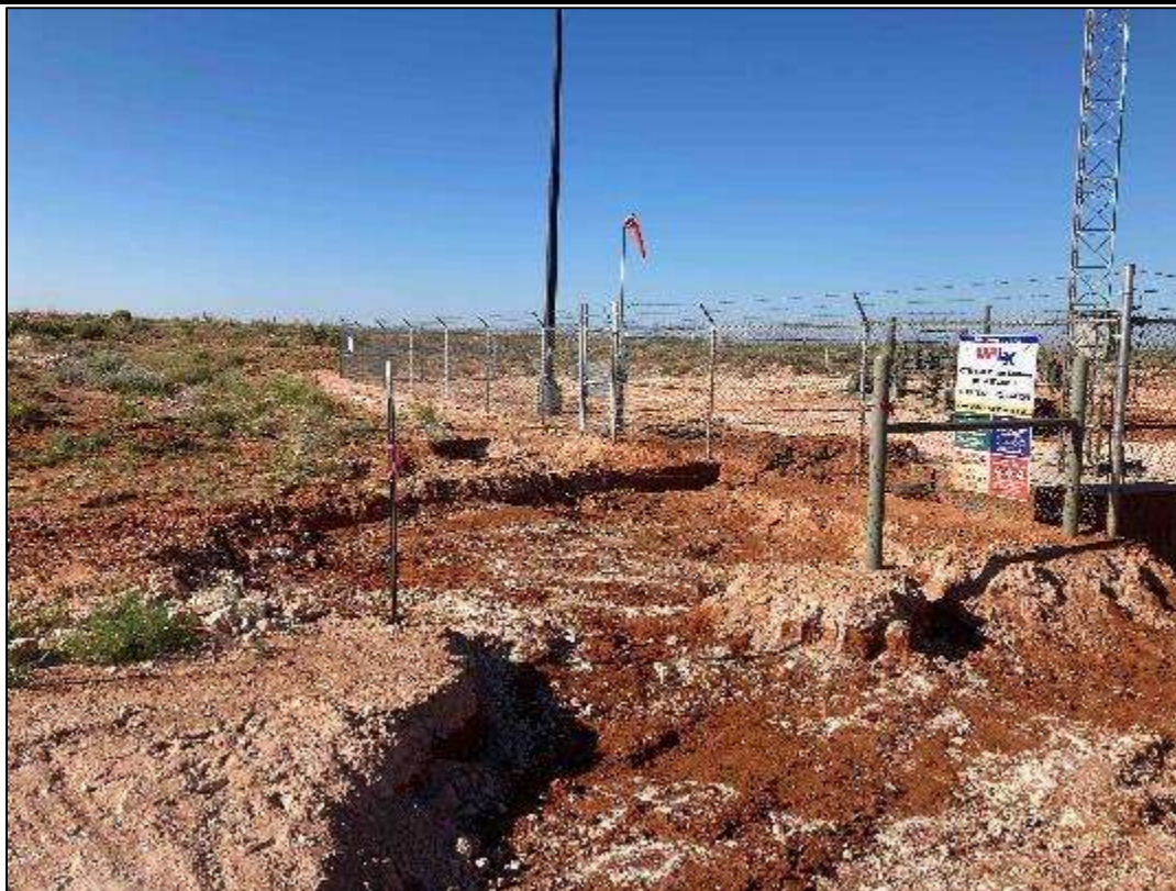
PHOTO 9: View of the excavated area facing southwest. 8/29/22
