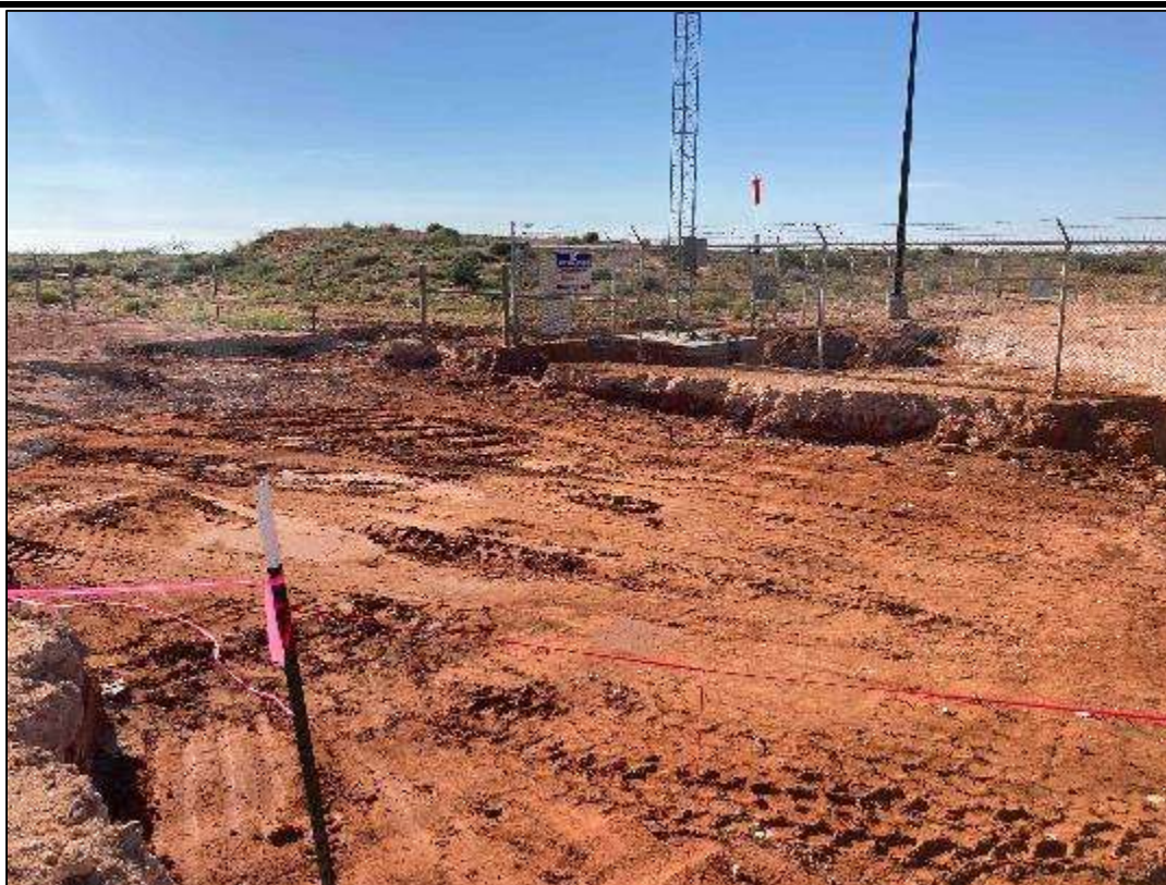
PHOTO 8: View of the excavated area facing southeast. 8/29/22
