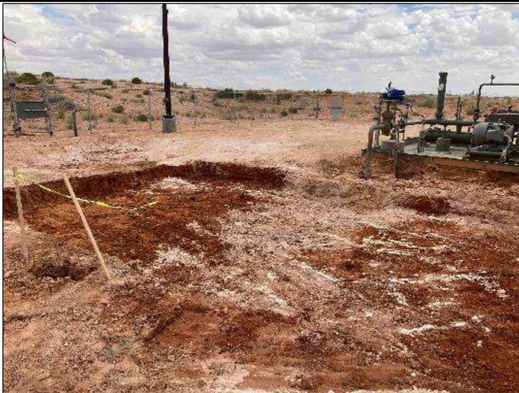
PHOTO 7: View of the excavated area facing southeast. 8/11/22
