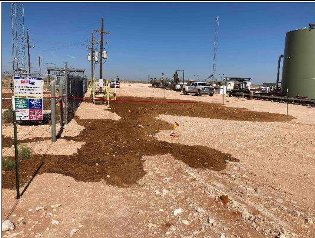
PHOTO 3: View of the impacted area facing west. 7/28/22
