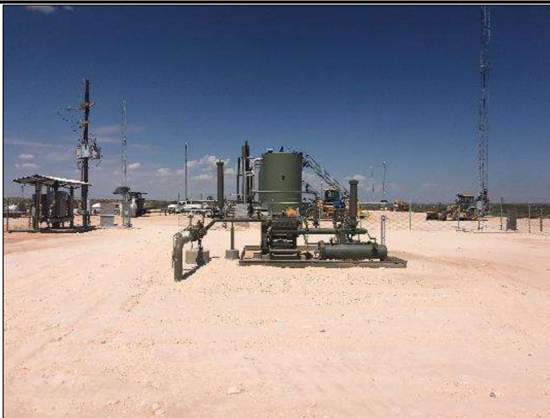
PHOTO 12: View of the remediated area facing north. 9/15/22
