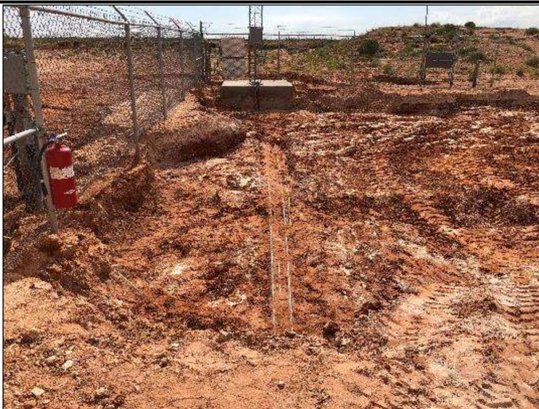
PHOTO 6: View of the excavated area facing east. 8/19/22
