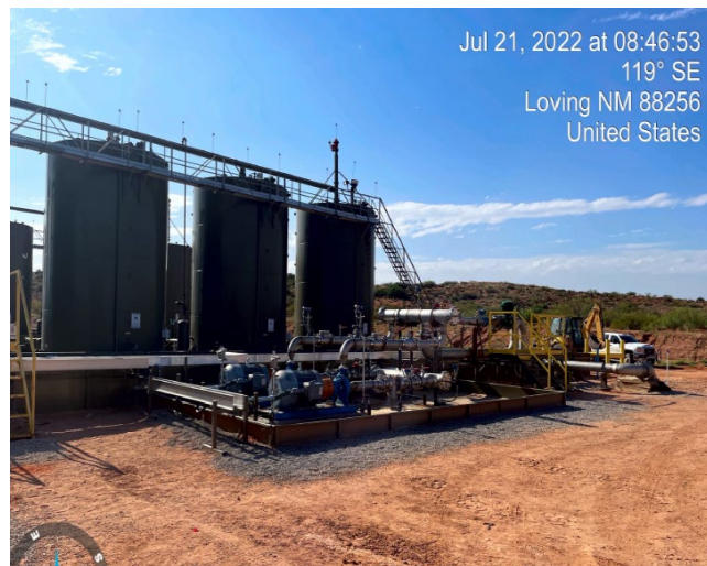
Photograph 4 Date:07/21/2022 Description: View of repaired containment following lateral delineation, facing southeast
