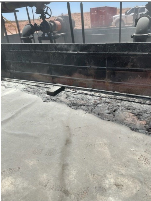
Photograph 1 Date:05/31/2022 Description: View of damage to the liner due to the fire, facing north
