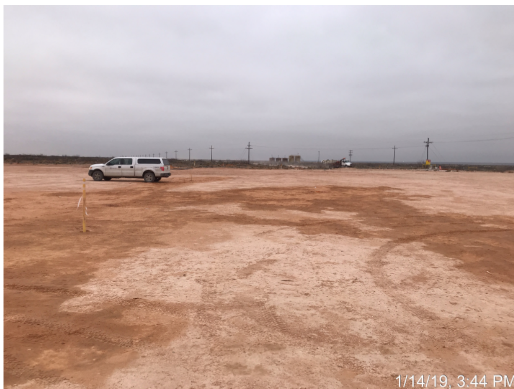
Area of AH-6 – View West
