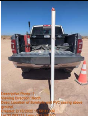
Viewing Direction: North
