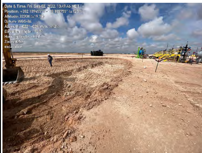
Photograph 4 Date: September 2, 2022 Description: Excavation Activities
