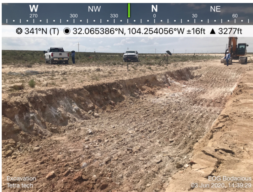
View of Remediation – View North/Northwest
