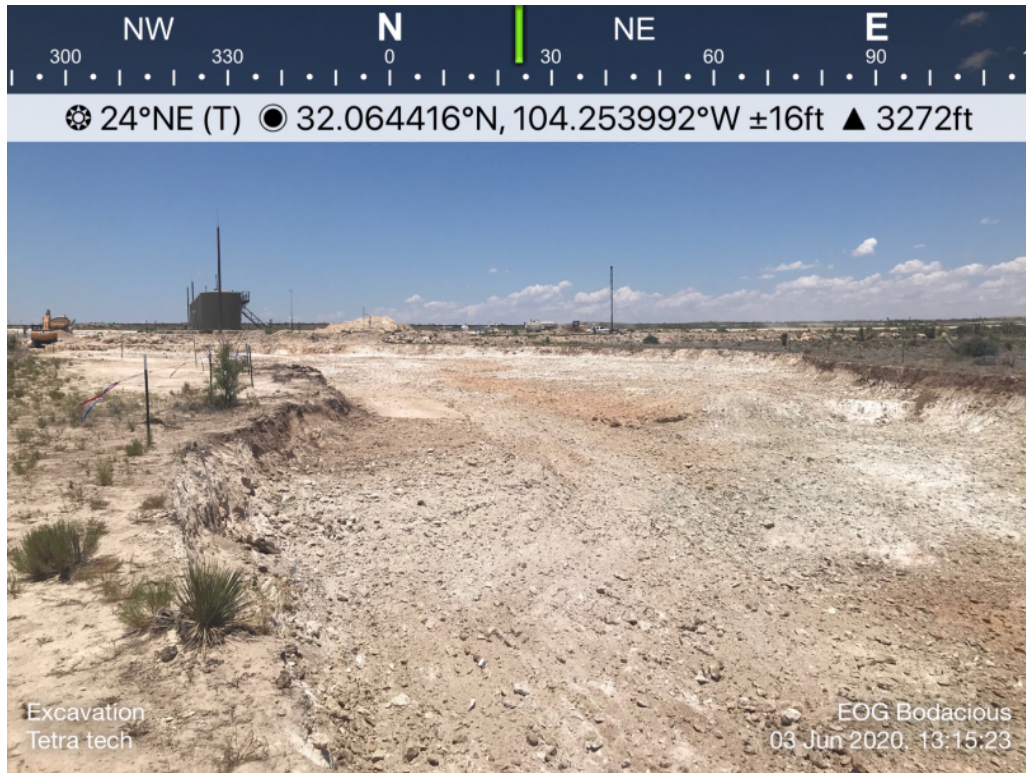
View of Remediation – View North/Northeast
