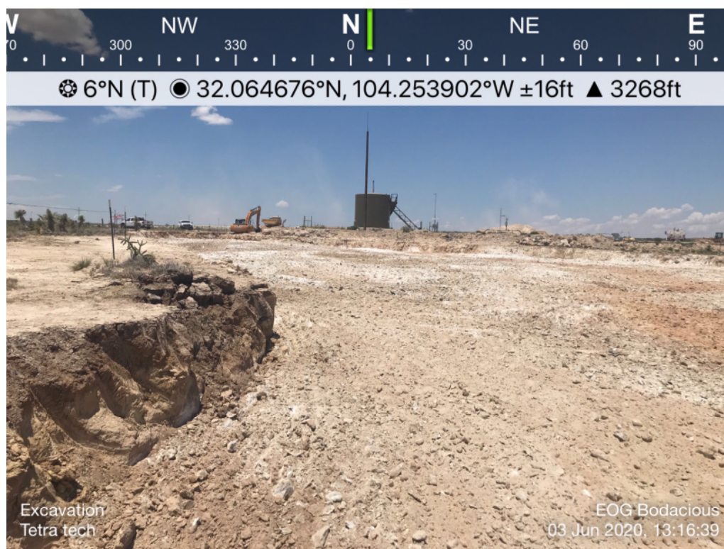
View of Remediation – View North
