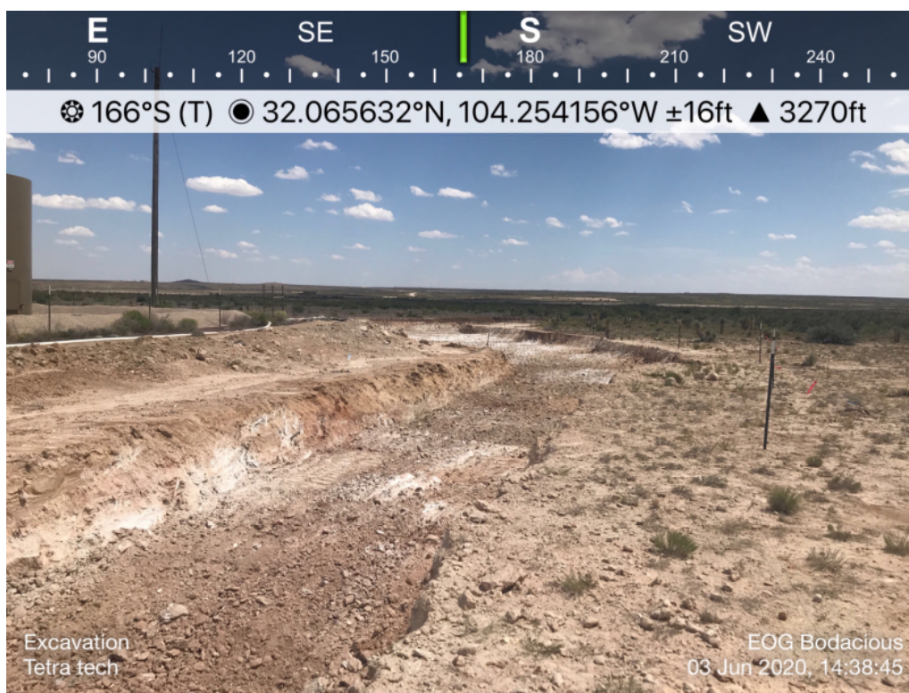
View of Remediation – View South
