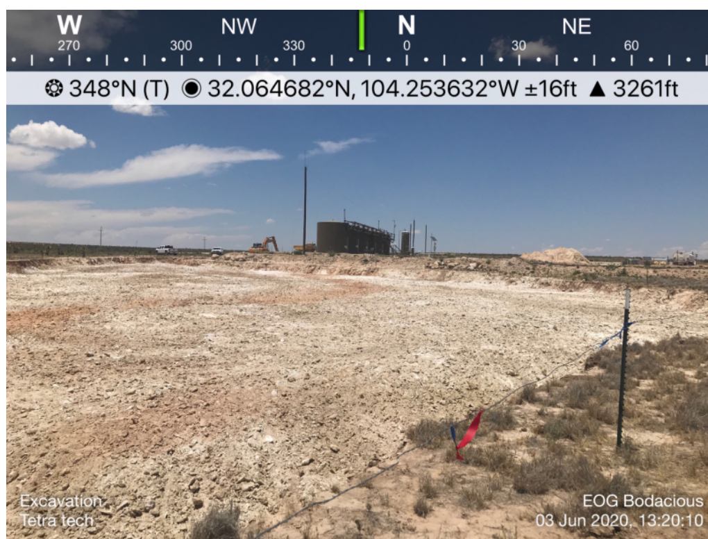
View of Remediation – View North
