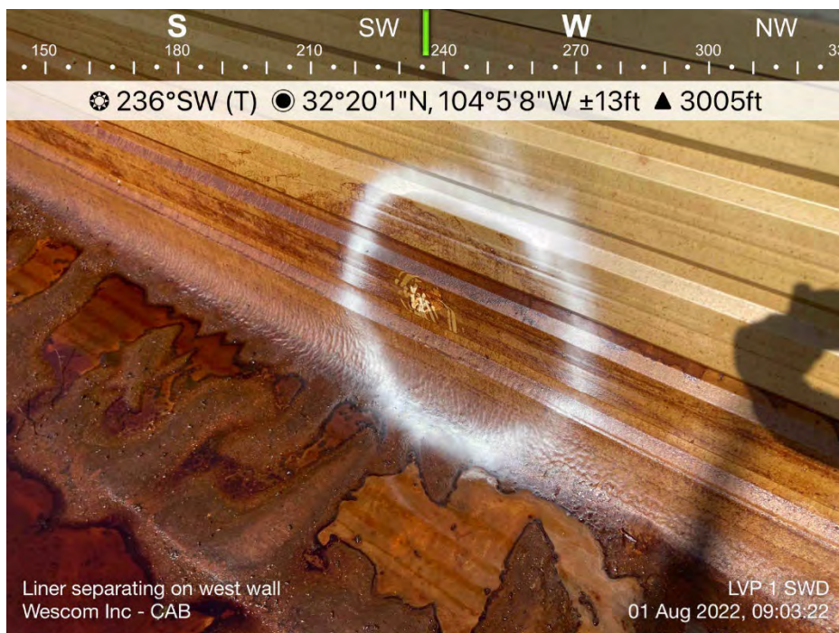
Liner peeling on West Wall
