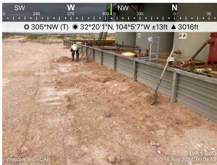
Potholing to Find Ground Wire – South Side
