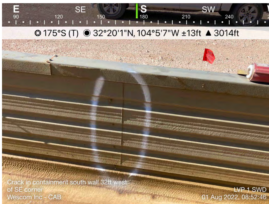
Crack in Containment Wall - Southeast Corner
