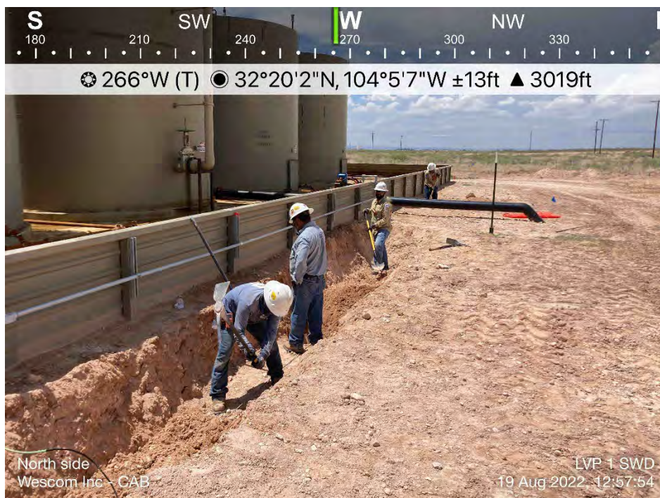
Hand Digging Over Ground Wire – North Side
