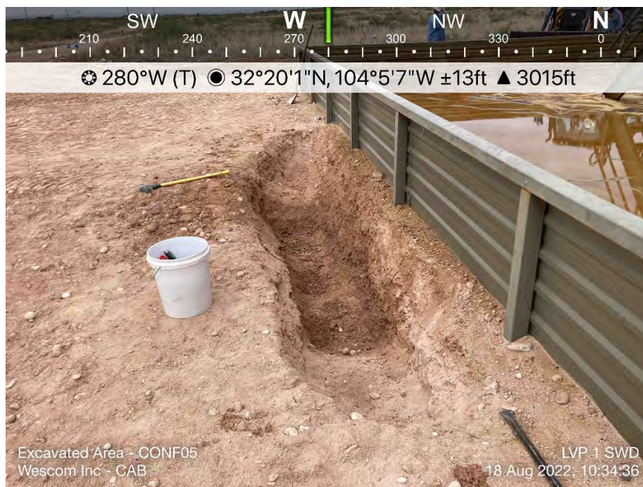
Excavation of Spill Area – Southeast Side (CONF05)
