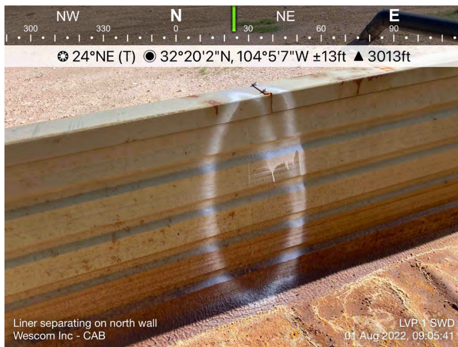
Crack in Containment Wall – North Side
