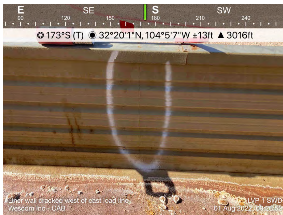
Crack in Containment Wall - South Wall
