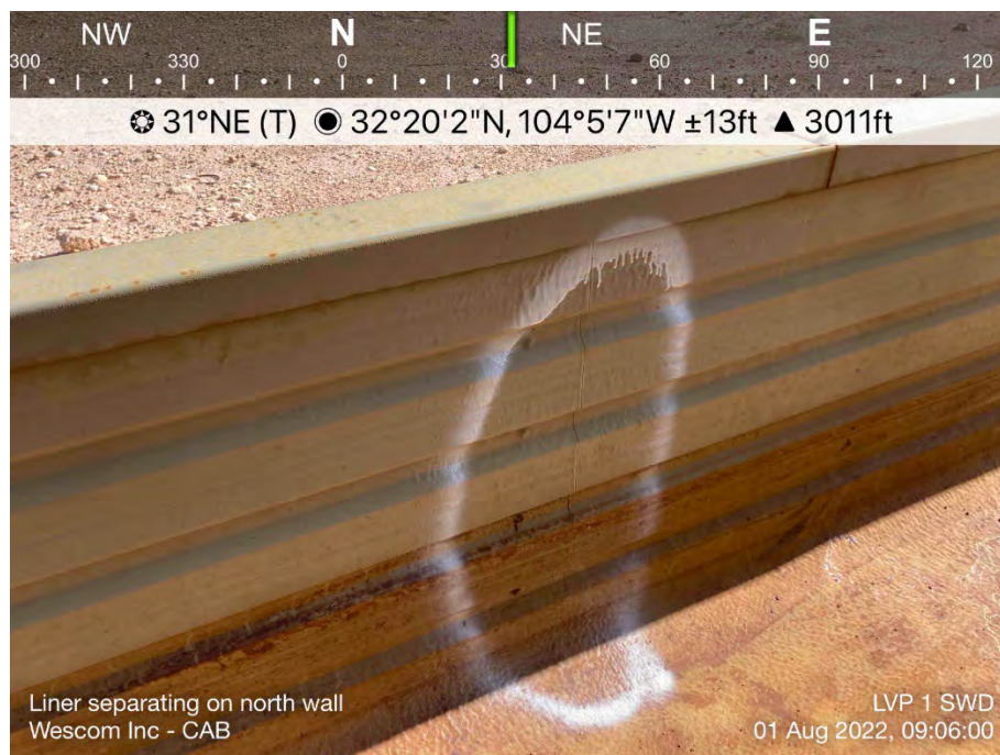
Crack in Containment Wall - North Wall
