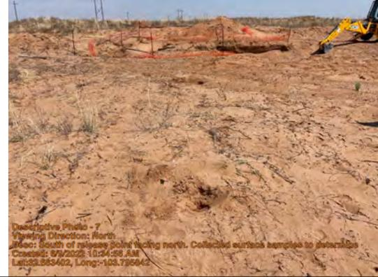
South of release point facing north. Collected surface samples to determine where to start boreholes.
