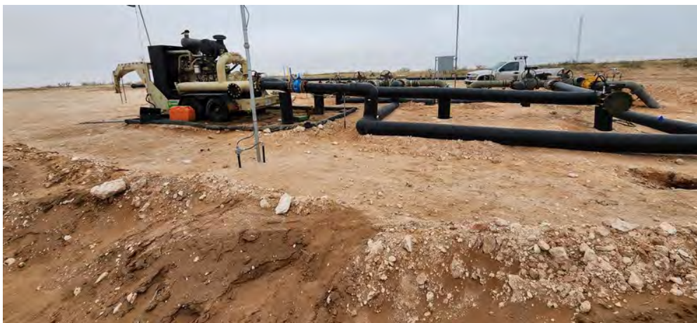
Figure 3: View of off-site production equipment along ROW at grids G-01, G-04 and G-05. The upper 0.5-feet of impacted material has been removed.
