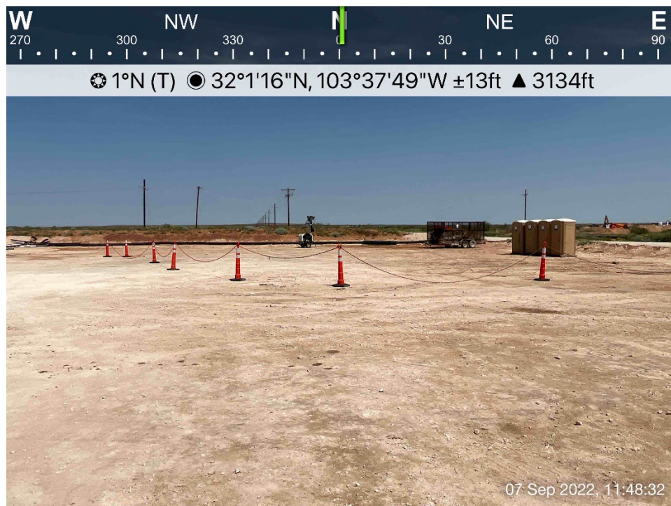
Impacted area viewing north, September 7, 2022
