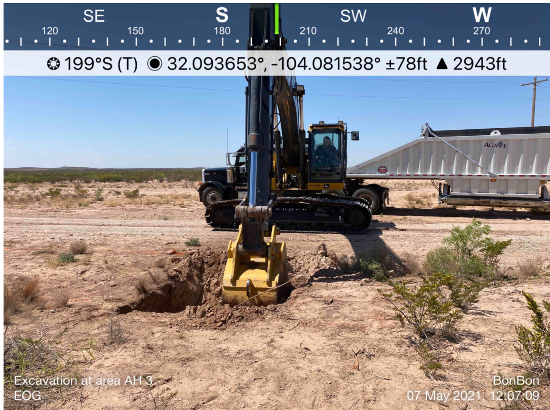
View of Remediation Activities – View South
