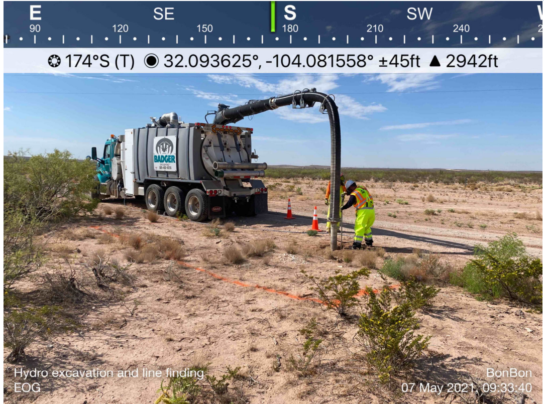
View of Remediation Activities – View Southeast
