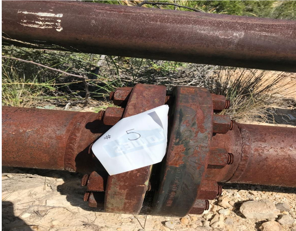
View East – Area of AH-5
