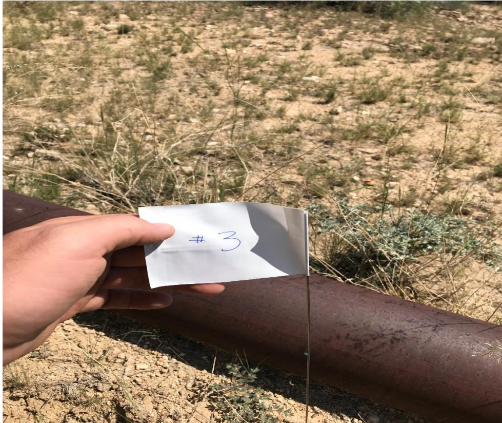
View East – Area of AH-3
