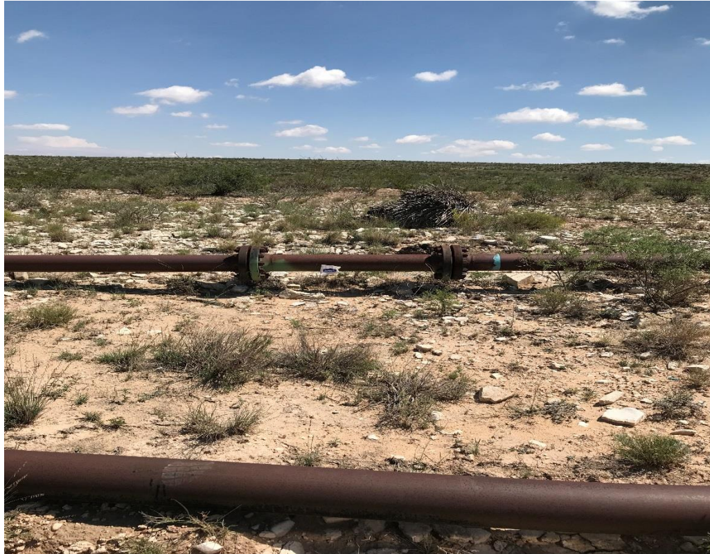
View East – Area of AH-11
