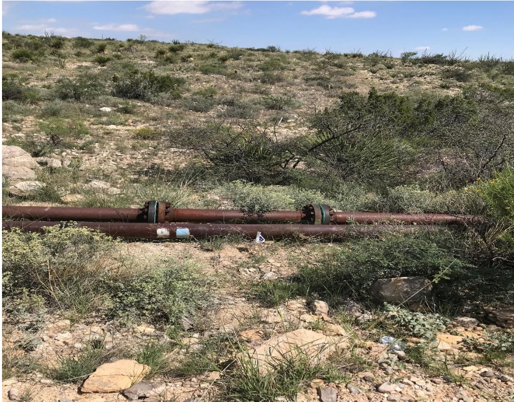
View East – Area of AH-1
