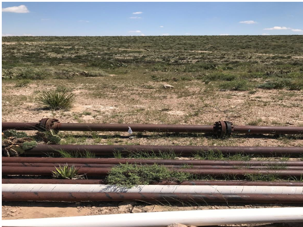
View East – Area of AH-6
