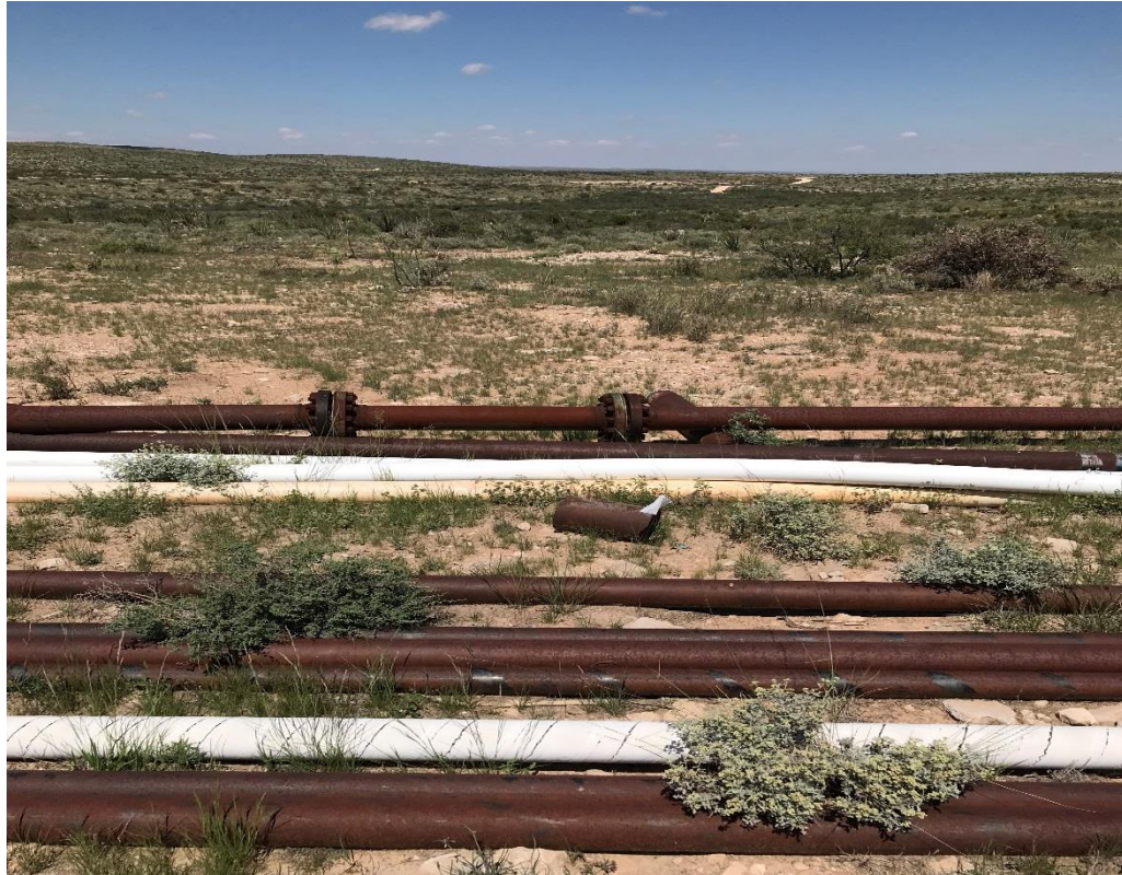
View North – Area of AH-9
