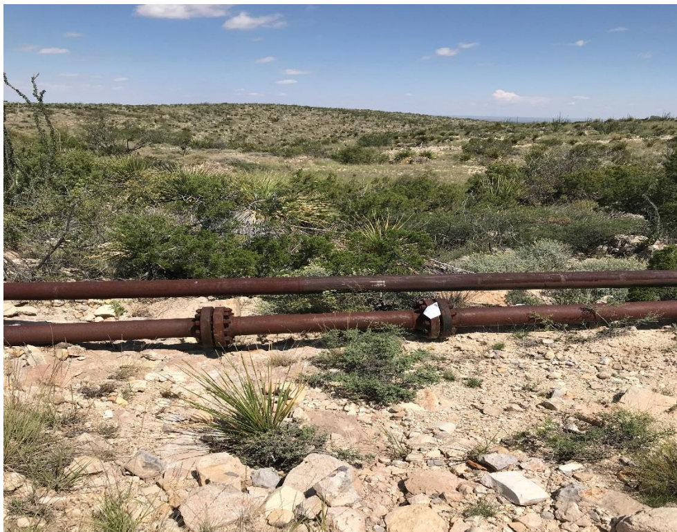
View North – Area of AH-4
