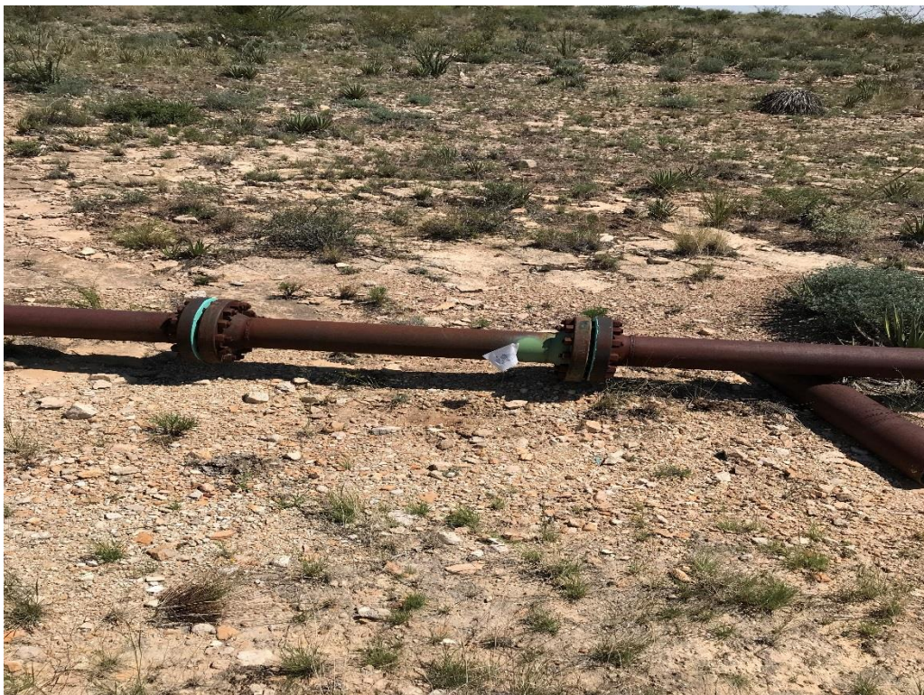
View East – Area of AH-2
