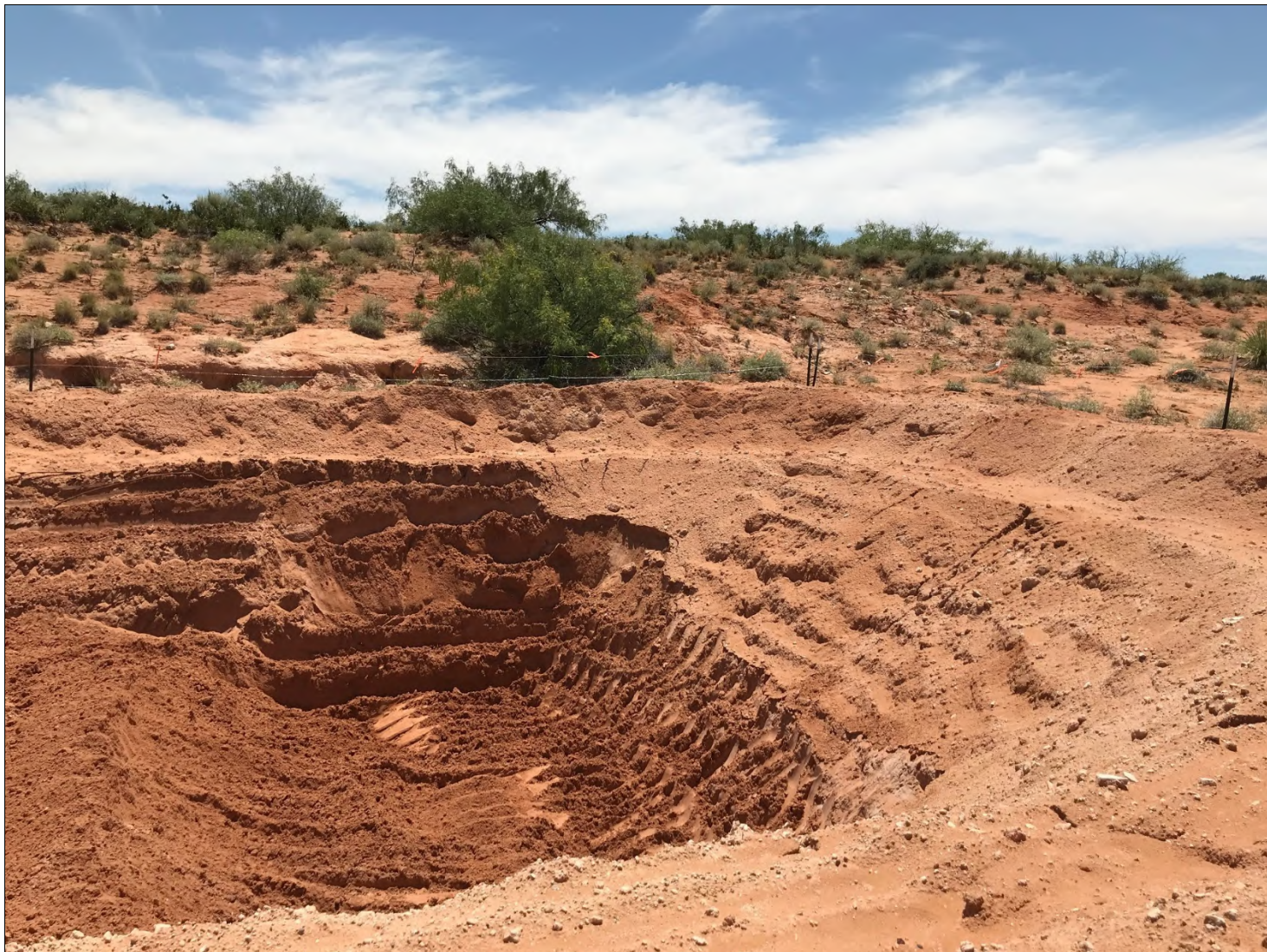
Eastern view of the final excavation.
