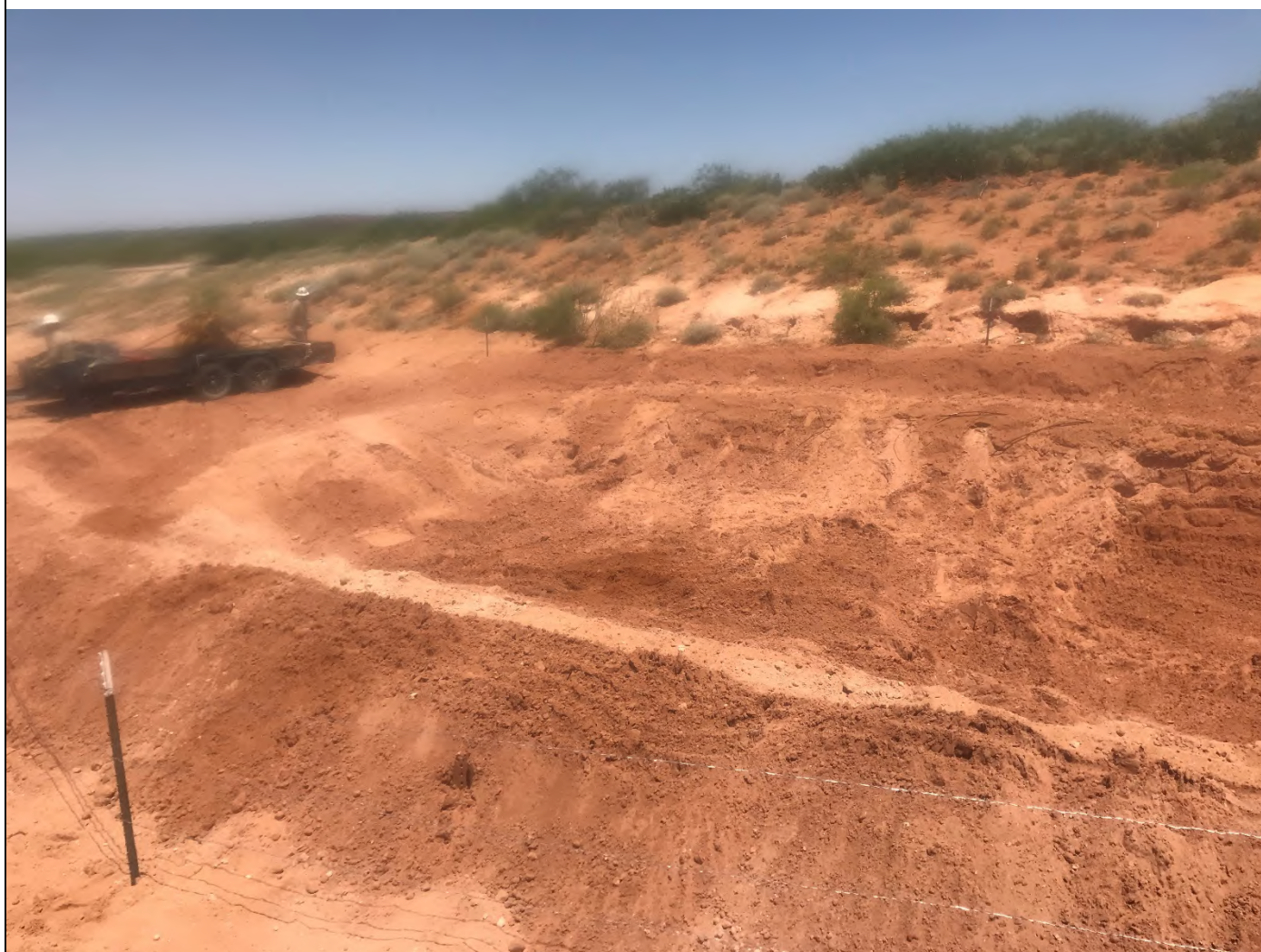
Northeastern view of the excavation.
