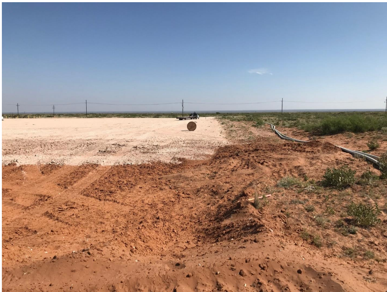
Northern view of release extent during preliminary soil sampling and site assessment.
