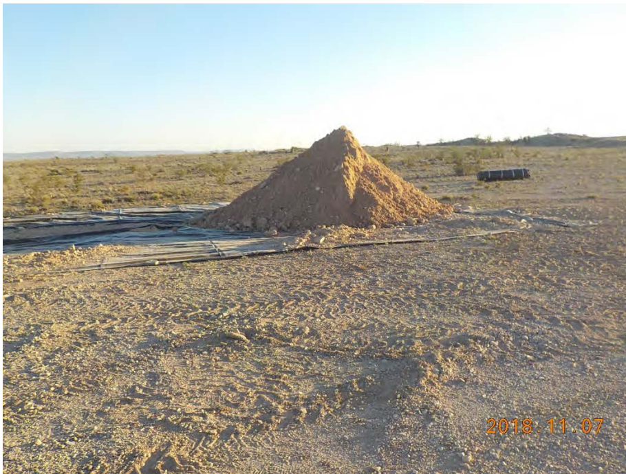
Typical view of excavated soil stockpile. View toward the south.
