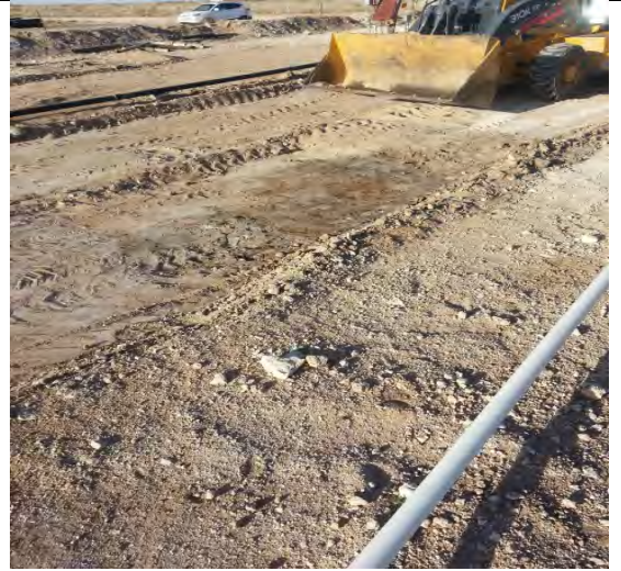
Impacted soil removal
