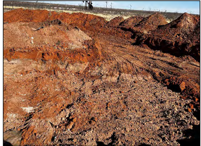
Photograph: 2 Date: 1/10/2023 Description: Excavation activities View: South
