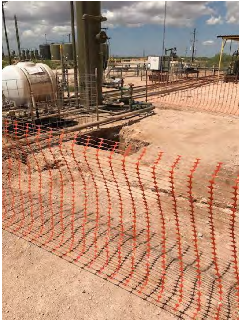
Fenced excavation near processing equipment.
